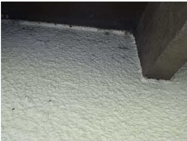
Wall top – sealed
