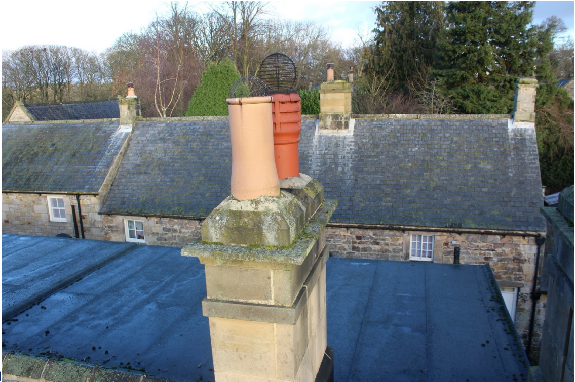
Figure 6: Existing chimney stack
