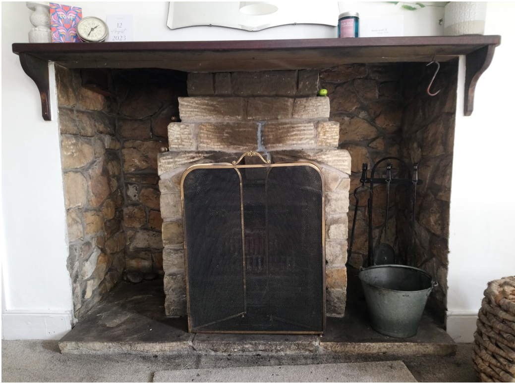
Figure 5: Existing coal fireplace and stone tile hearth
