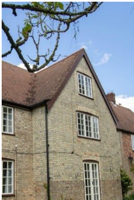
Fig. 2a: South front of house with projecting wing
