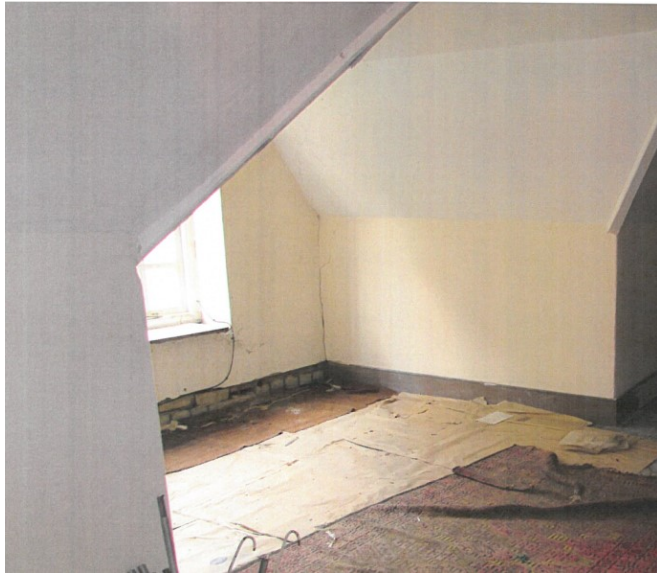
Fig. 2b: Second floor central bedroom in projecting rear wing.
