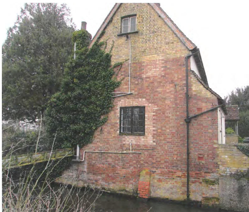
Fig. 22 East Elevation – C20 whites on Victorian reds on C18(?) revetment
