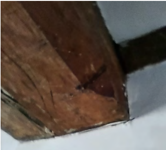
Fig 18: ceiling beam detail on Ground Floor
