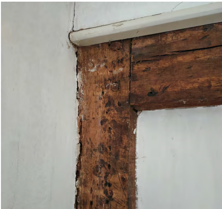
Fig 20 – Junction of principal corner post and FF beam in Dining Room
