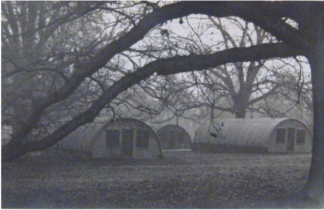
Fig. 14: Another row of Nissen Huts within the Station Hospital complex (1944)
