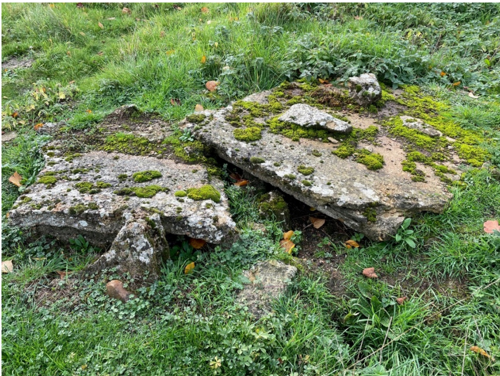
Fig. 23: Partially removed concrete footings showing composition of site footings
