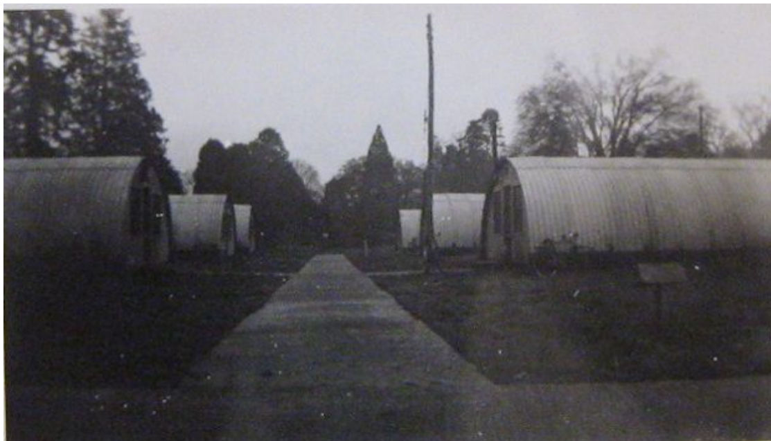
Fig. 13: Row of Nissen Huts within the Station Hospital complex (1944)
