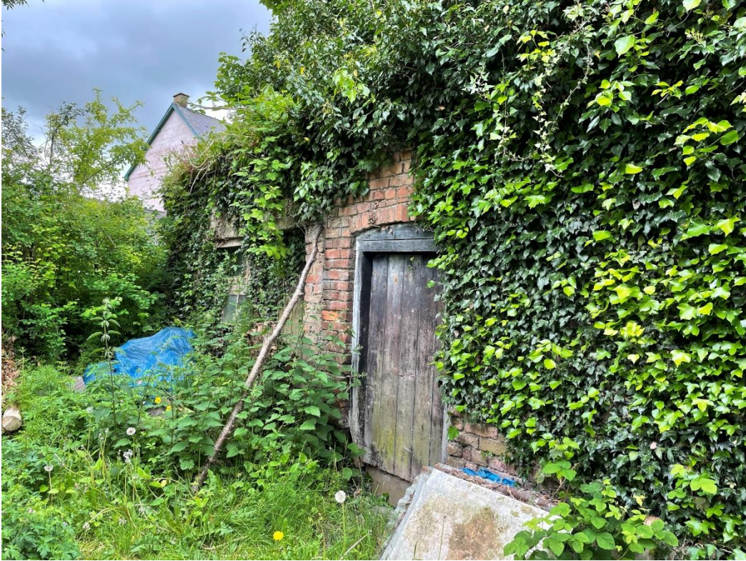
Photo 3. Northeast elevation with windows and side door
