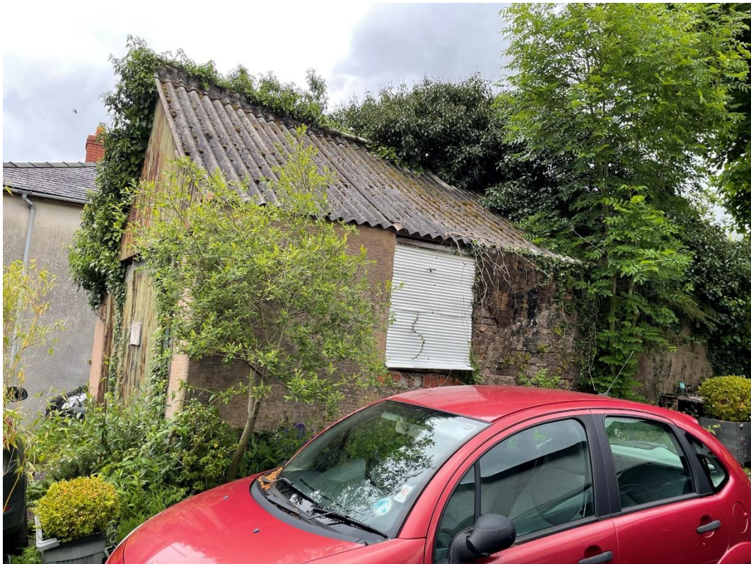
Photo 6. Southwest elevation with metal covered window
