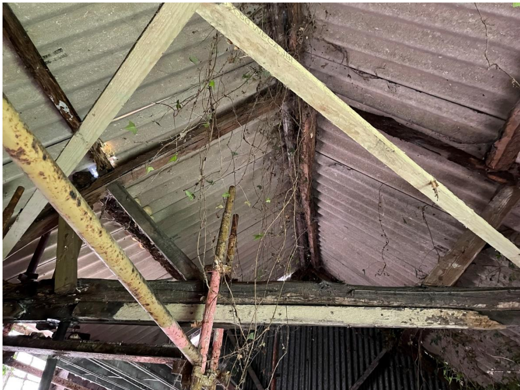
Photo 12. Interior showing scaffolding holding up the roof
