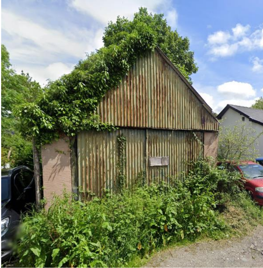
Photo 1. The Garage – northwest elevation
