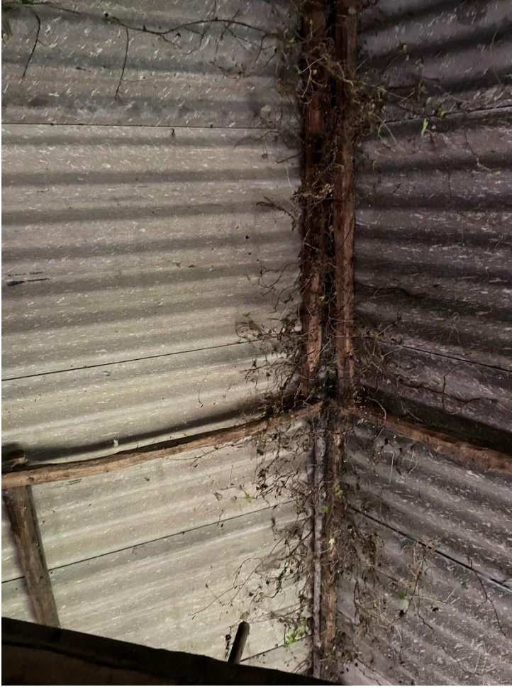
Photo 11. Interior roof structure
