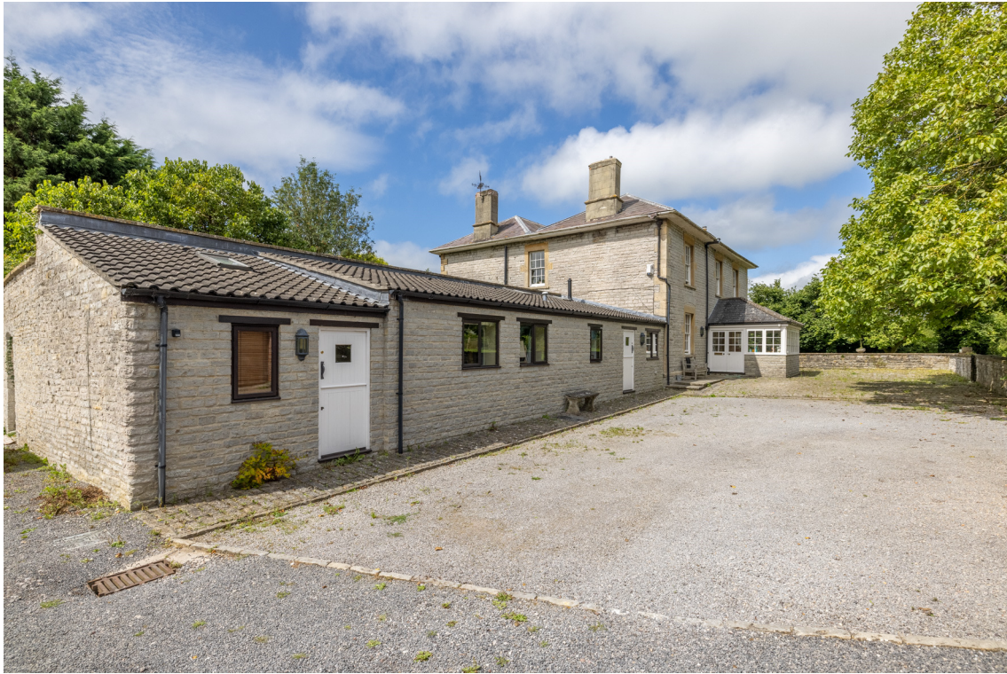
Rear of the house from the lane entrance
