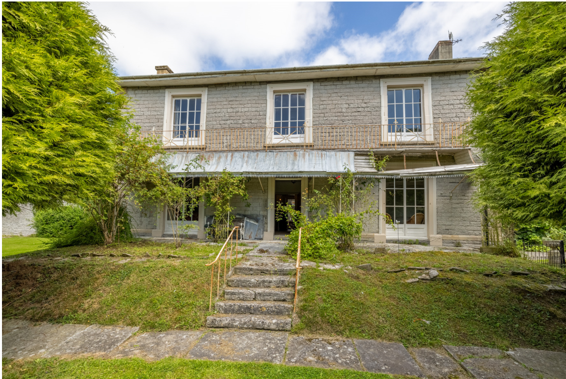
South west elevation (the two trees have now been felled)
