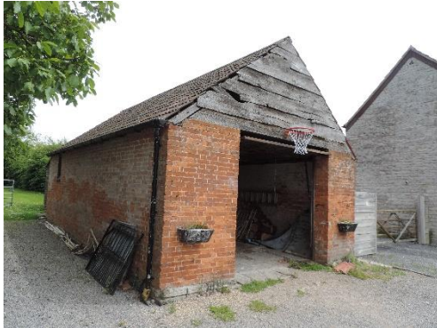
Plate 9: Example of Damaged Ridge Tile
