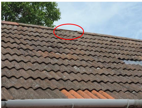
Plate 9: Example of Damaged Ridge Tile
