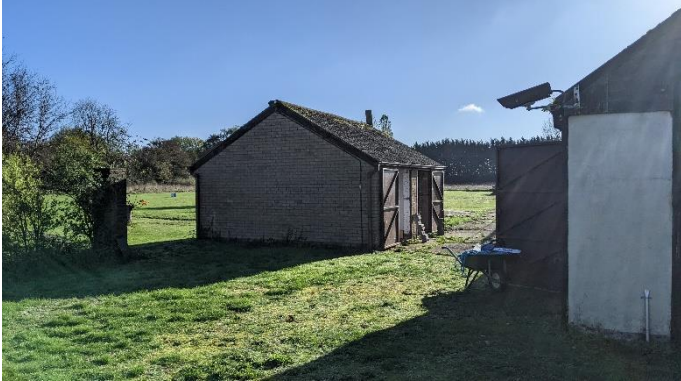
Photo 3 Building B1 – N and W elevations
