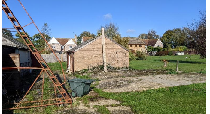
Photo 4 Building B1 south gable end
