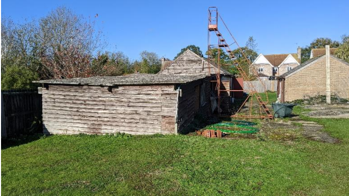
Photo 5 Building B2 South and east elevations
