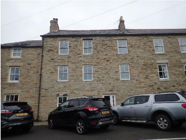
From the north, note open access windows
