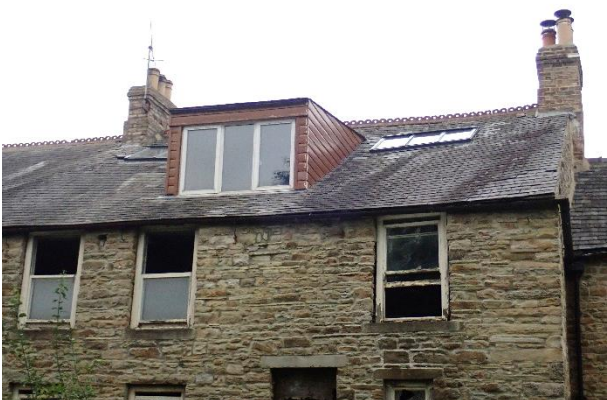
Roof of the north aspect
