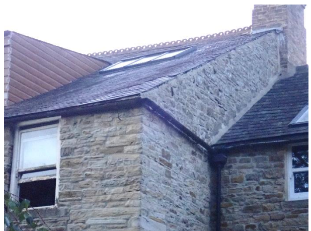
West gable showing raised slate – to be retained as at present
