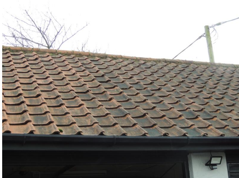
Photo 11: Showing tight seal to roof tiles
