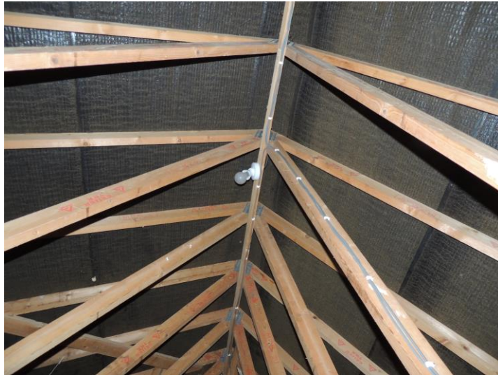
Photo 8: Showing roof construction
