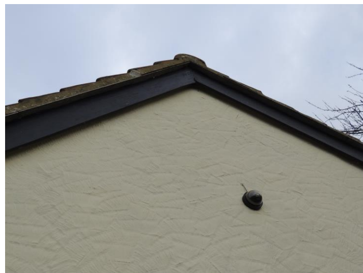
Photo 10: Showing tight seal to gable wall
