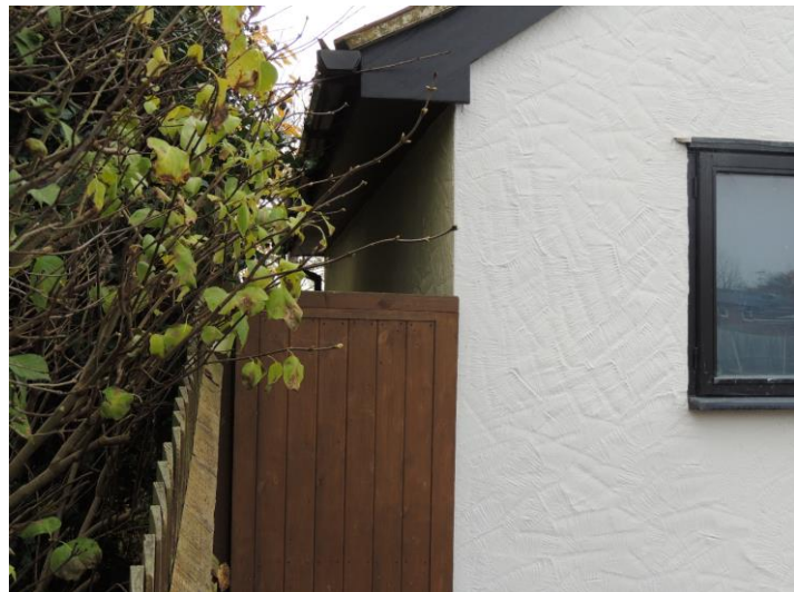
Photo 4: The southern elevation is obscured by the boundary fence and vegetation
