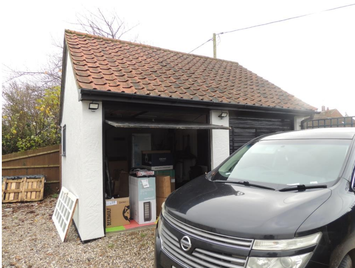
Photo 1: Northern elevation. The proposal is for an upper floor to the building
