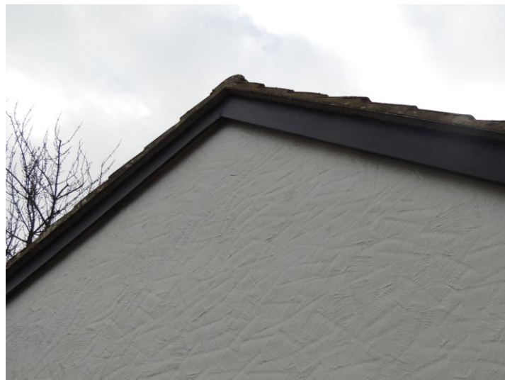
Photo 9: Showing tight seal to gable wall
