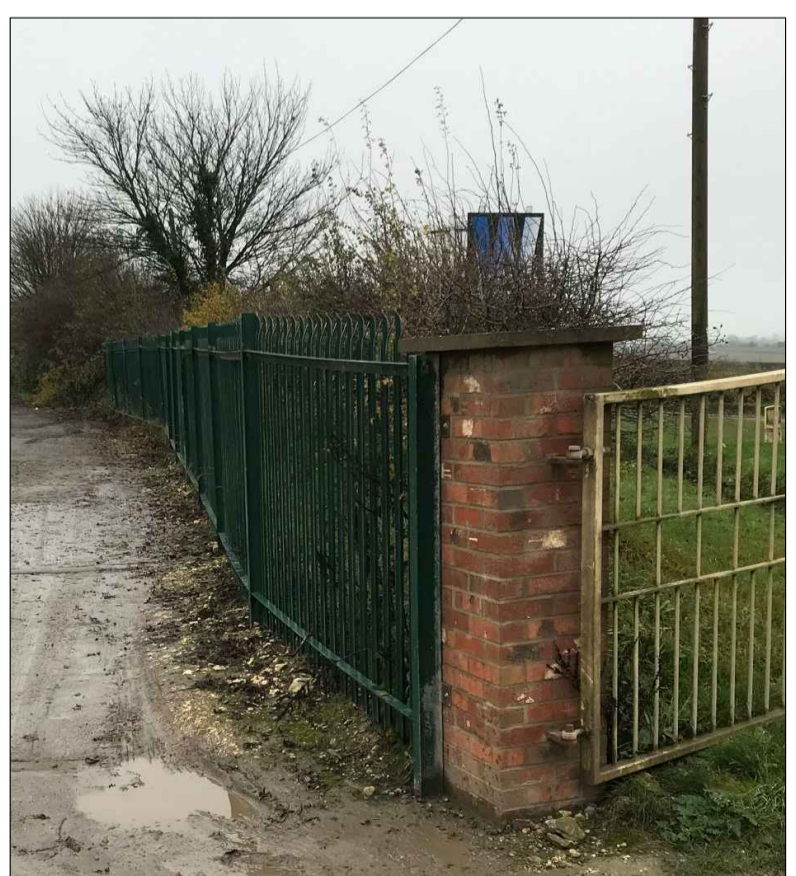
Existing Palisade Fence
