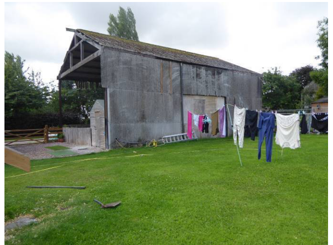
Northern asbestos clad elevation of the Dutch barn with surrounding amenity grassland.
