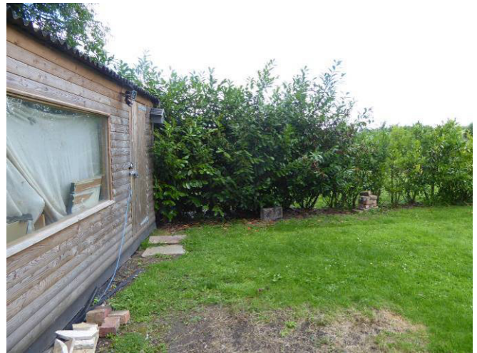
Wooden garage with corrugated roof on the sites western boundary. Bird boxes are present on the northern and southern ends of the eastern elevation.
