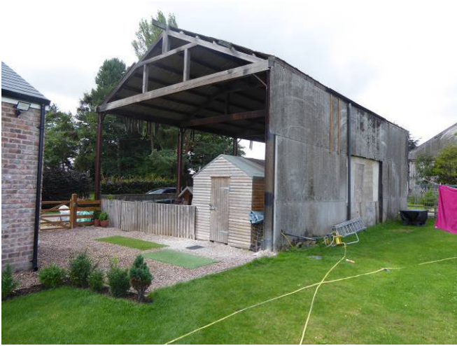
Dutch barn showing open east elevation and asbestos clad northern elevation.
