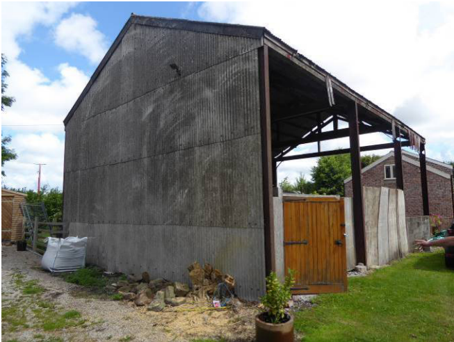
Dutch barn showing asbestos clad western elevation and open southern elevation.
