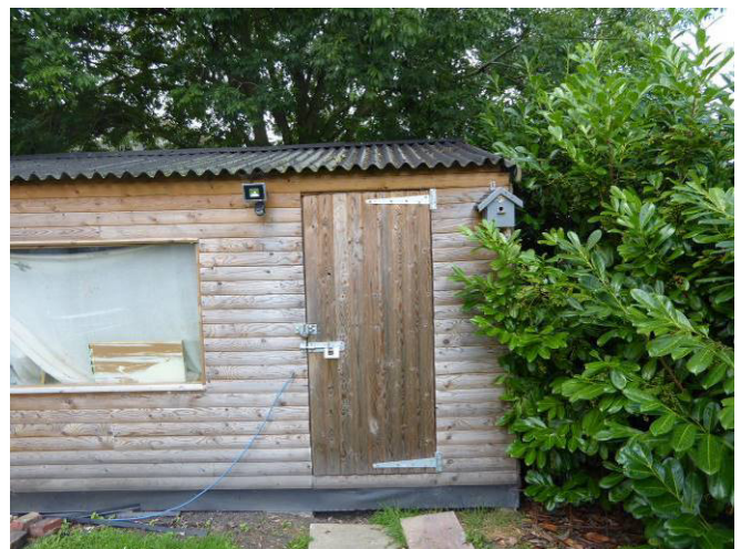
Wooden garage with corrugated roof on the sites western boundary. Bird boxes are present on the northern and southern ends of the eastern elevation.
