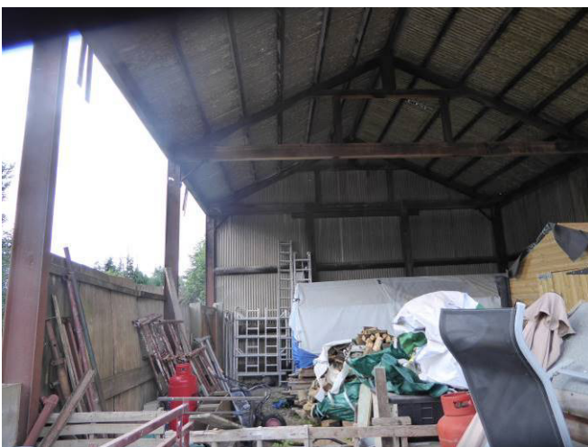
Internal area of barn showing wooden truss roof structure.
