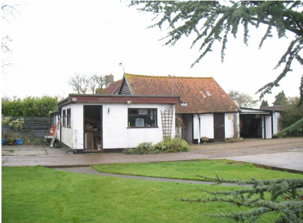
Part of the collection of outbuildings. Barn in the centre. Tack room closest. To the right the collection of garages to be rebuilt as a carport.
