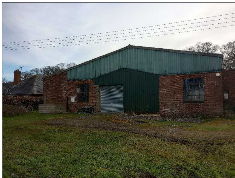
Figure 2.4: View of rear elevation of the building
