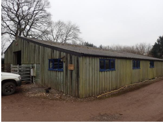
Figure 1. The northern and eastern elevations of the storage barn
