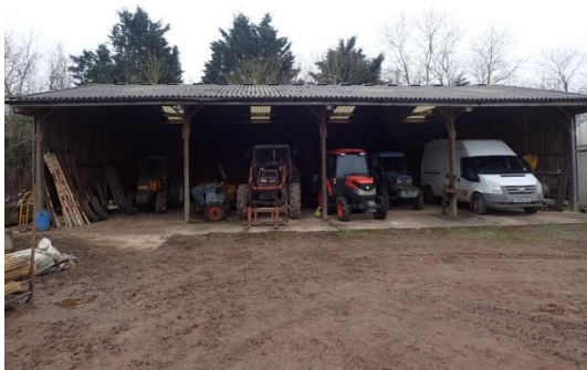
Figure 3. The eastern elevation of the tractor barn
