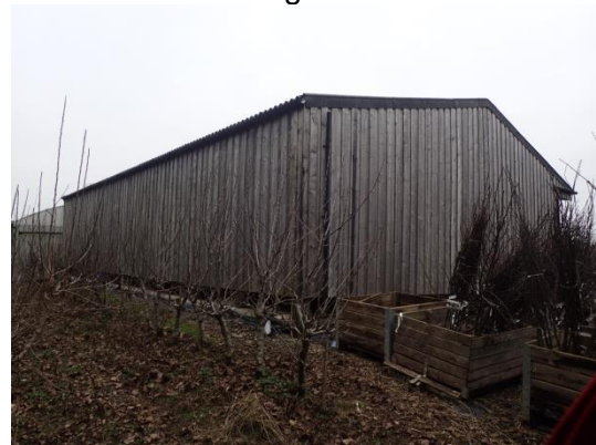
Figure 4. The western and southern elevation of the tractor barn
