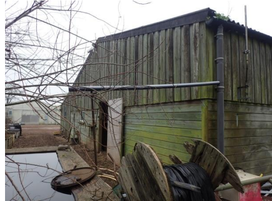
Figure 2. The western elevation of the storage barn
