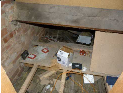
Photo 16. Small loft void
