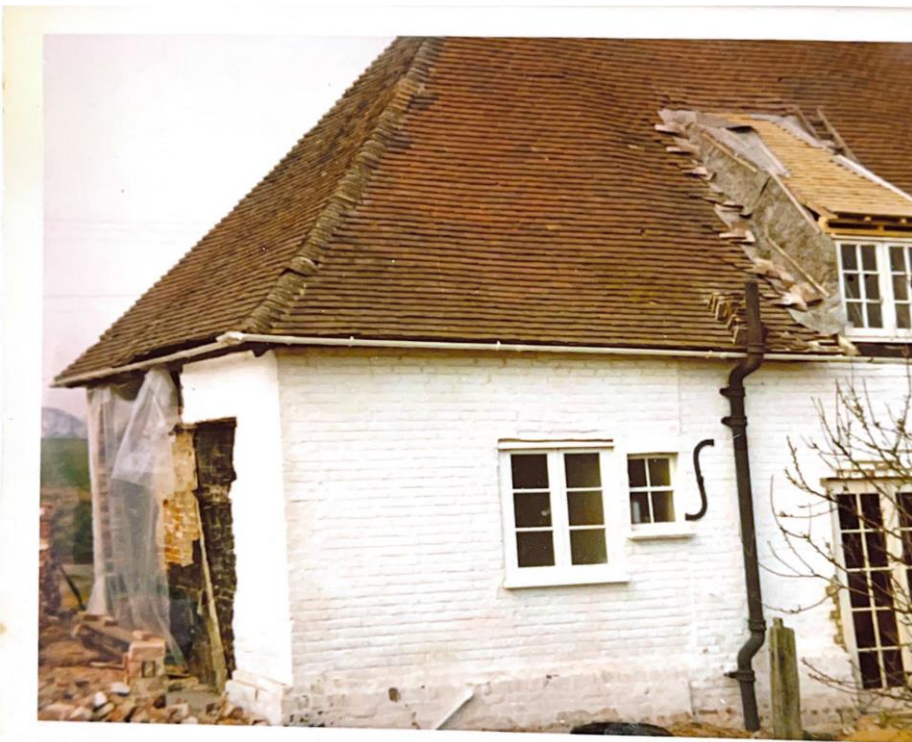
Above: Rebuilt side elevation
