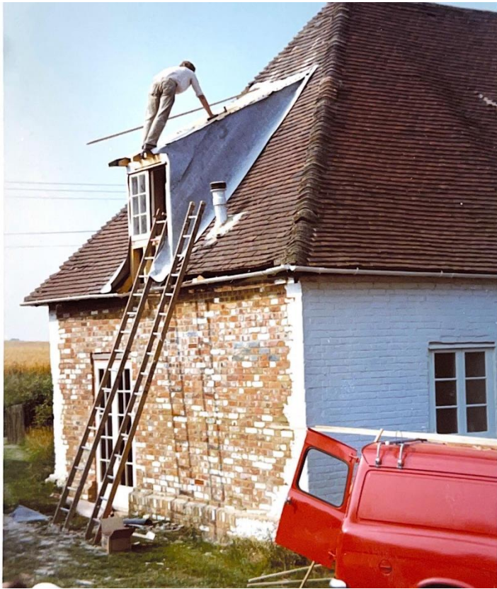
Above: Rebuilt side elevation
