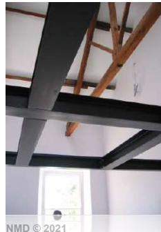
structure of mezzanine exposed
