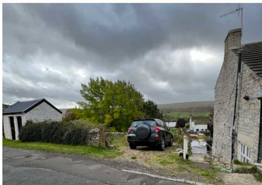
realign existing opening - with drystone wall
