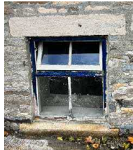
North elevation small casement WINDOW 009 - 012
