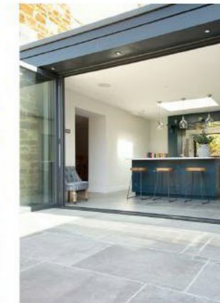
Aluminium projecting roof edge
