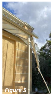
Figure 4 – Damage to Glass Canopy
