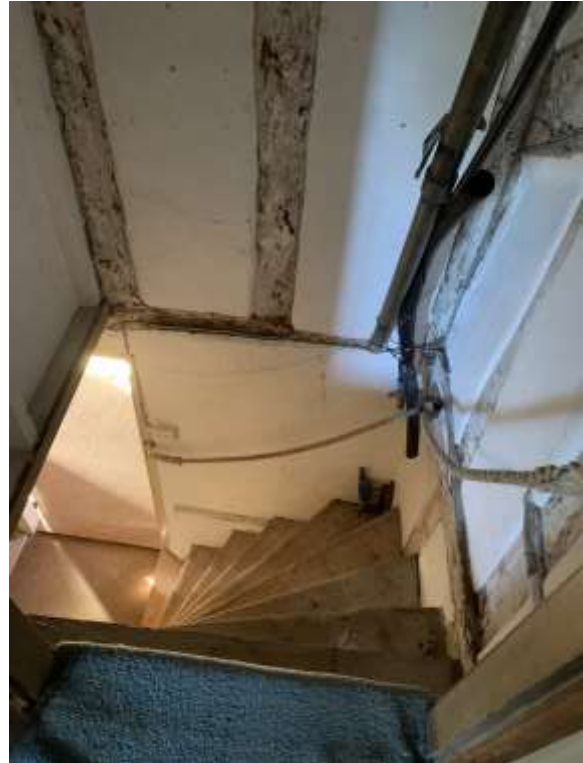
TWO OF THE STAIRS TO BE RETAINED & BOARDED OVER FOR SAFETY
