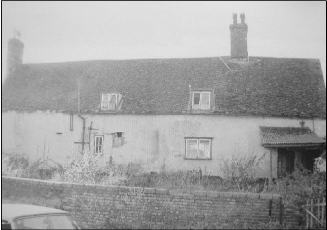
Fig .33 Mill House (c.1981)
