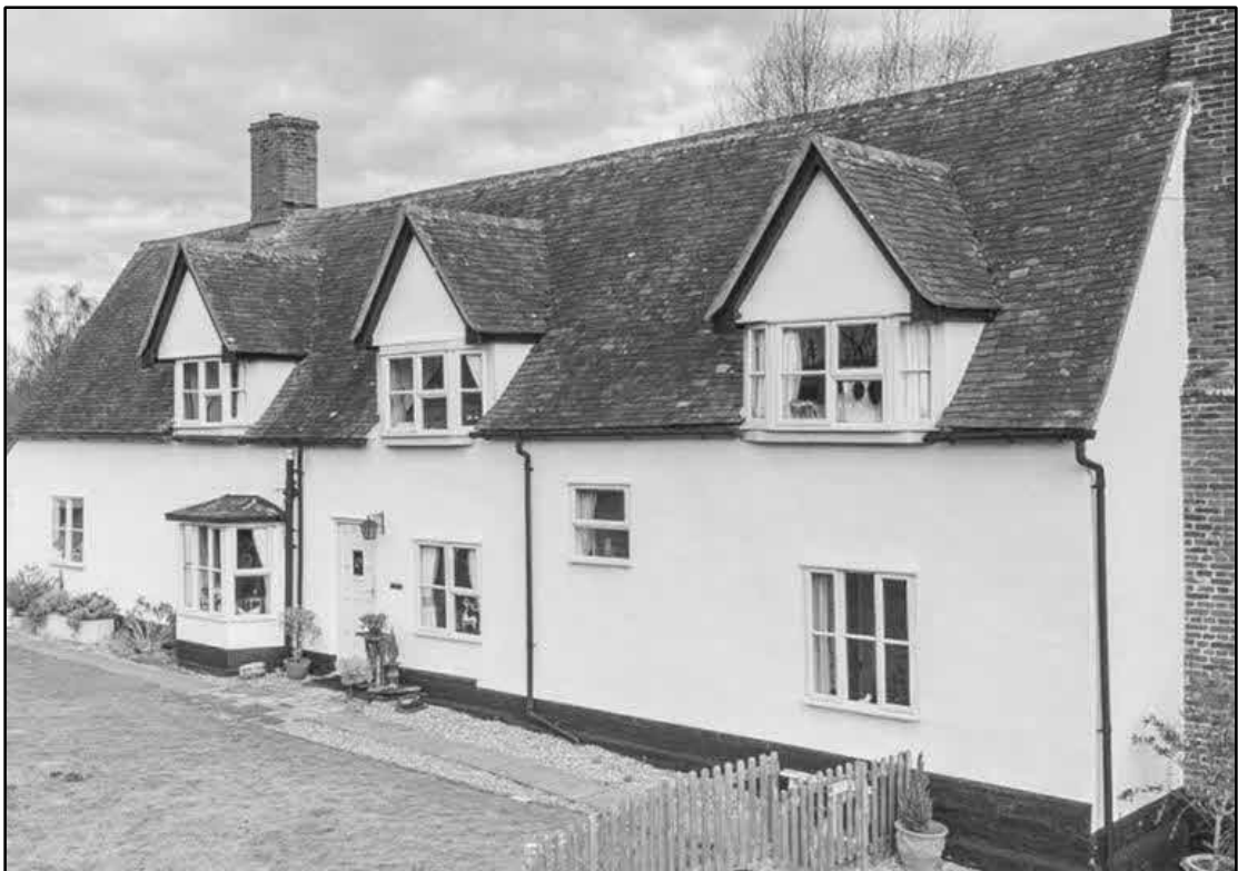
Fig.39 Mill House as restored in early 1980s
