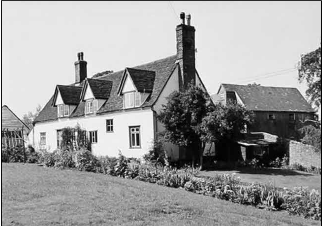
Fig .31 Mill House and Badley Mill (c .1966)
