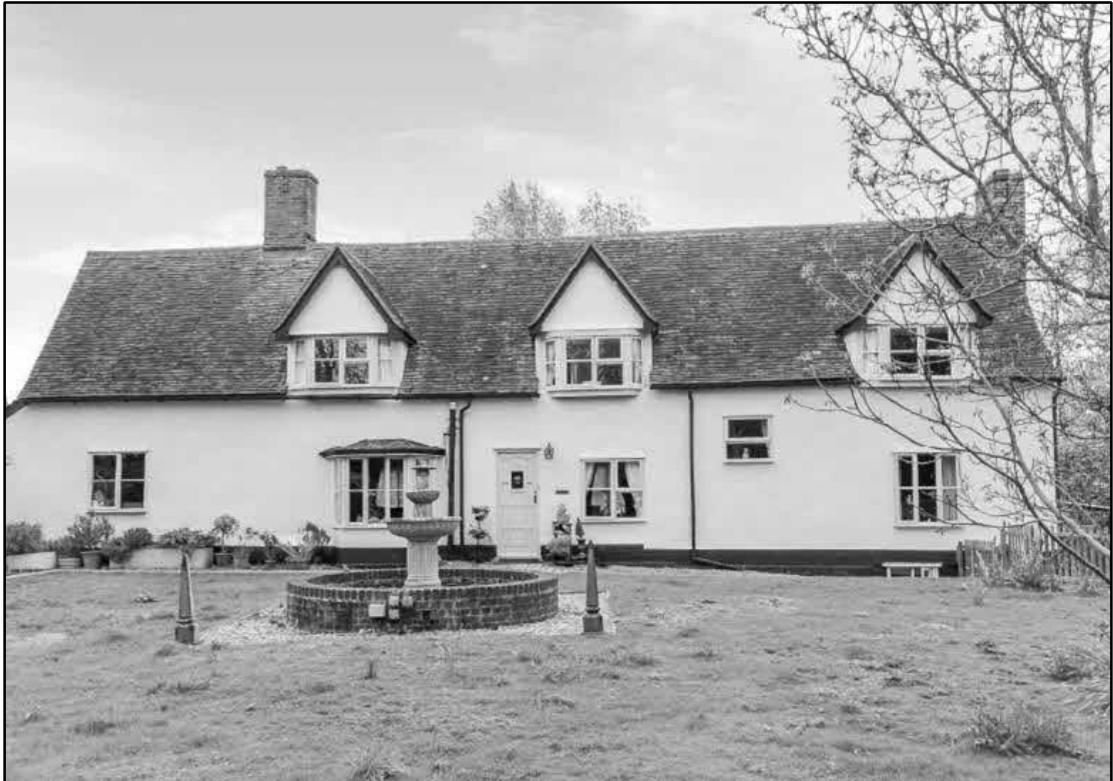
Fig .38 Mill House as restored in early 1980s
