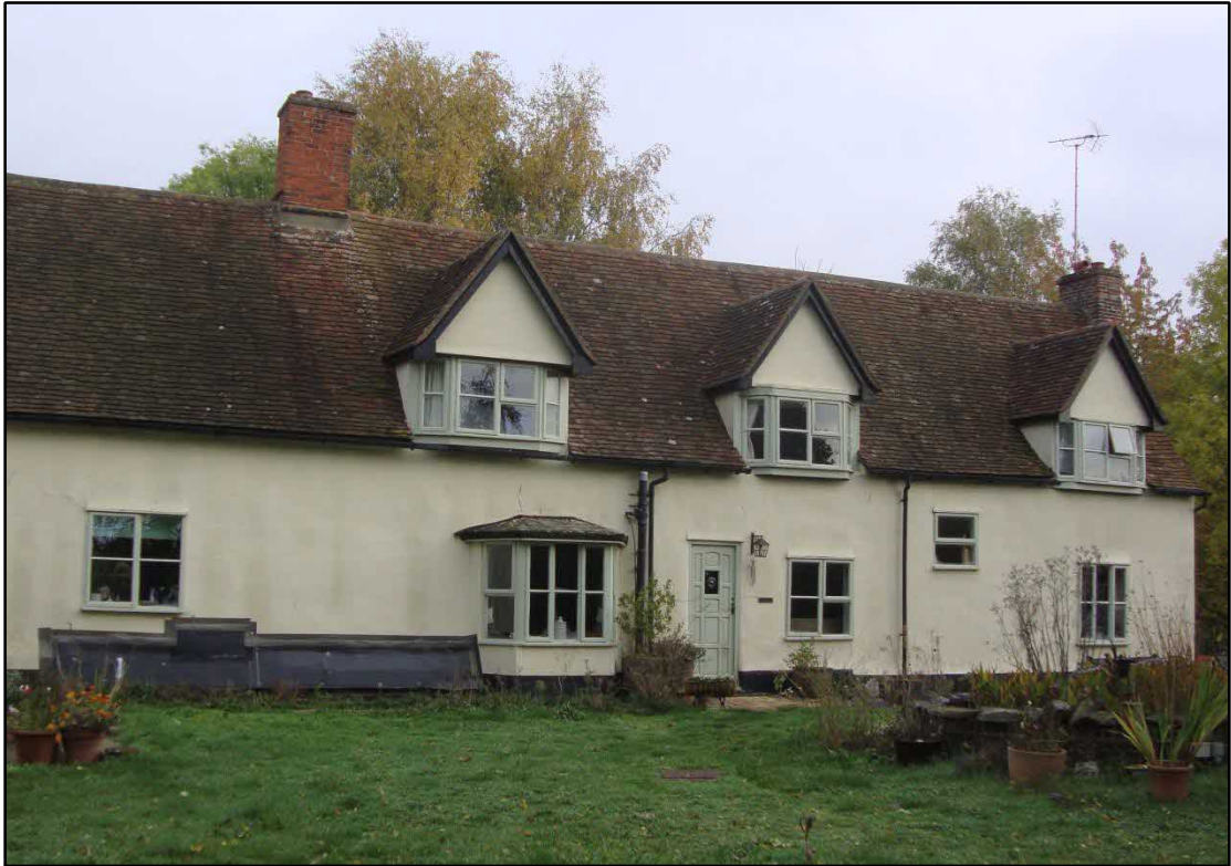
Fig.1 Mill House (south-west)
