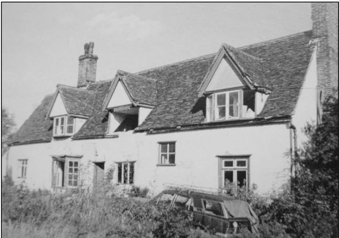
Fig .32 Mill House (c.1981)
