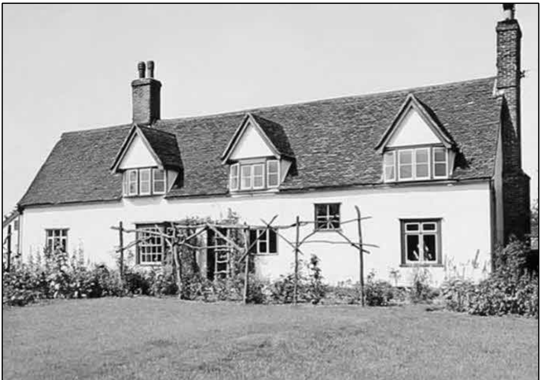
Fig.30 Mill House (c.1966)
