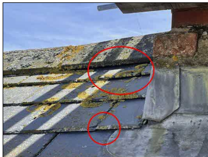
Plate 11. Examples of gaps under roof and ridge tiles
