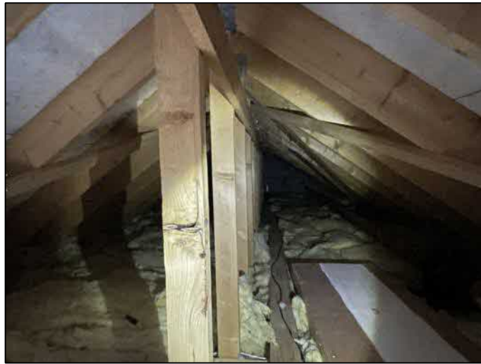
Plate 8. Loft 4 above two-storey extension
