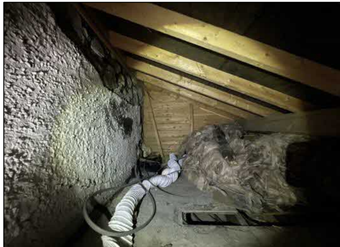
Plate 7. Loft 3 above north-eastern lean-to extension
