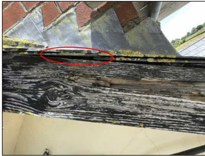
Plate 13. Gaps in timber cladding on lean-to extension (red arrows) and location of bat droppings in gap between cladding and frame (green arrow)
