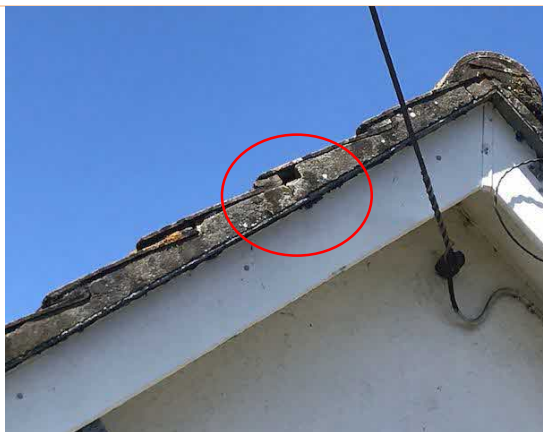
Gaps under tiles suitable for use by bats
