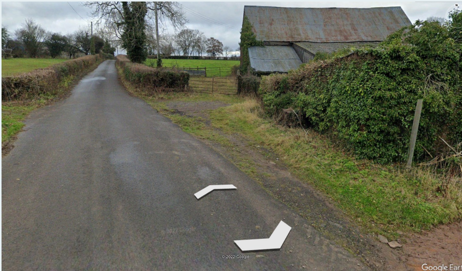
Road to Grosmont looking North
