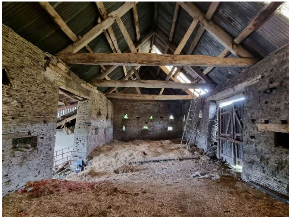
Barn interior looking west
