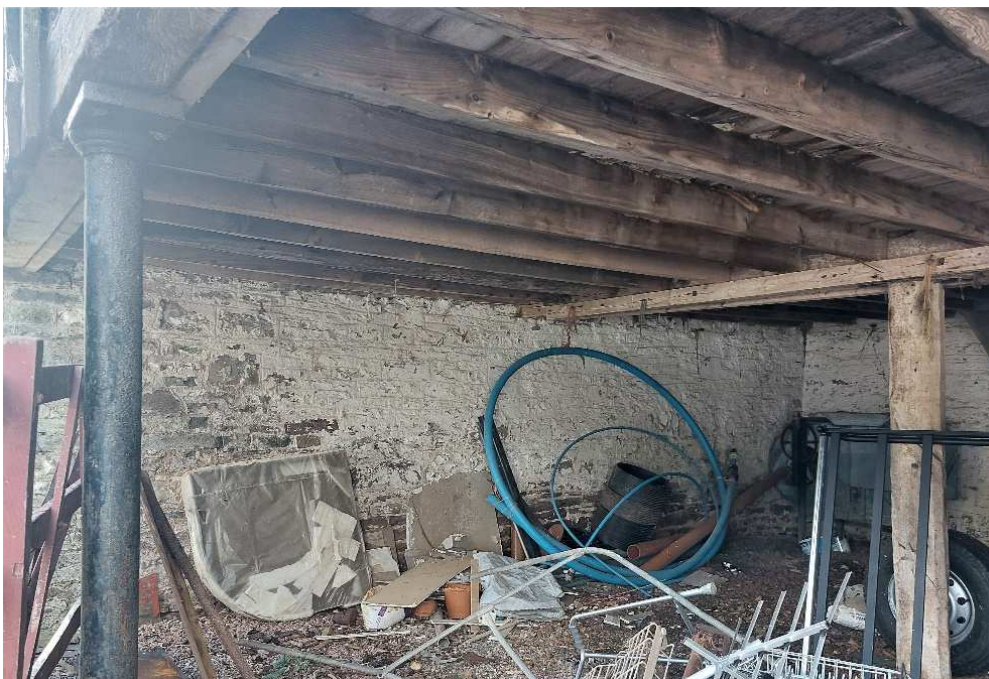
7. The iron post supporting the front of the cart shed
