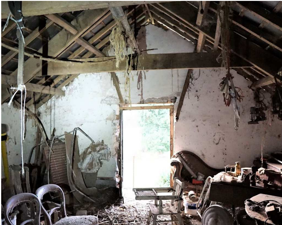
16. The lime washed interior of the Cider House loft
