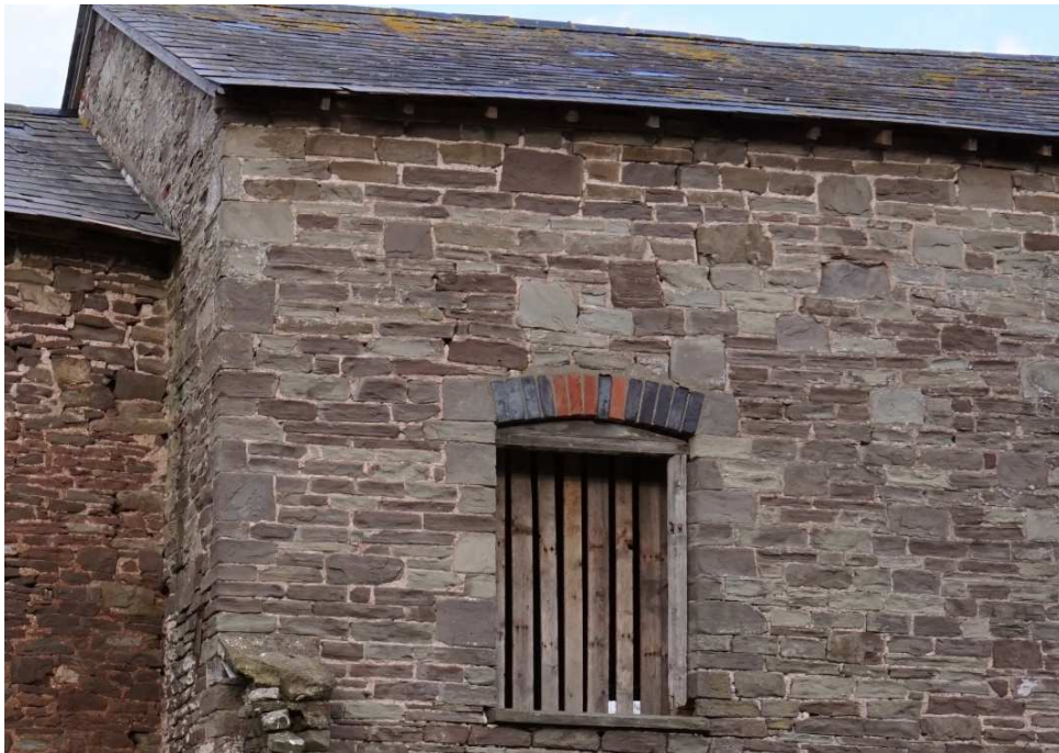
13. The south wall of the Cowhouse
