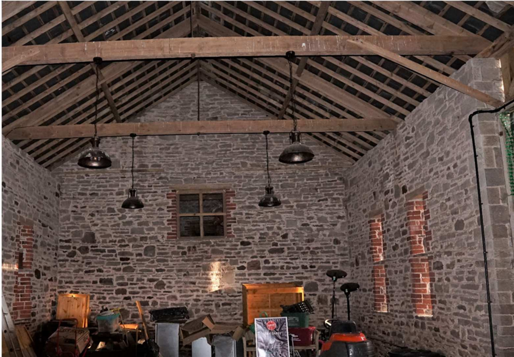
11. The interior of the threshing barn
