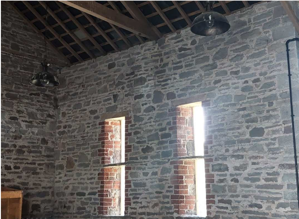
9. Interior view of the south wall.
