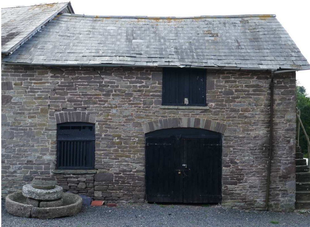
14. The frontage of the Cider House has had extensive rebuilding
