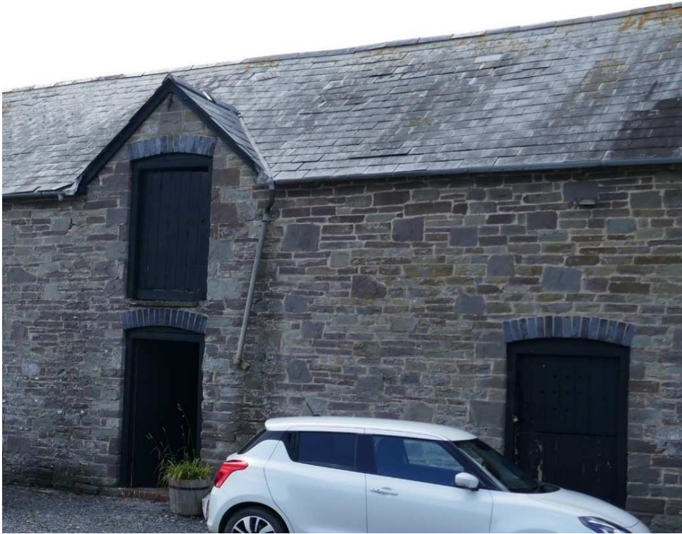
12. The north wall of the Cowhouse
