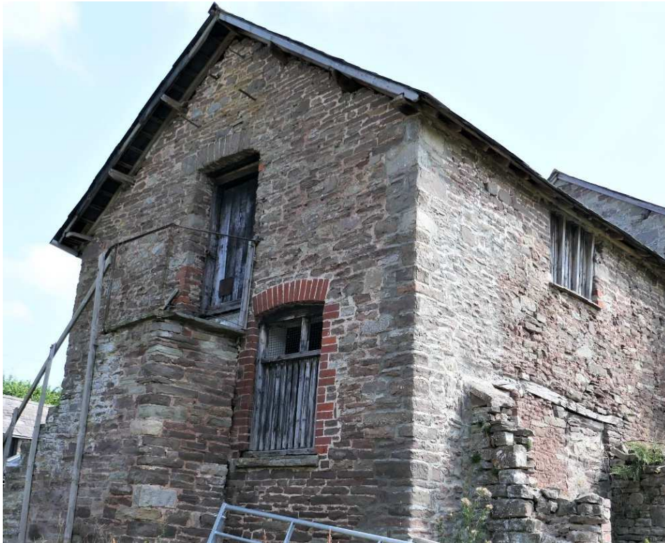
15. The west gable wall with external steps
