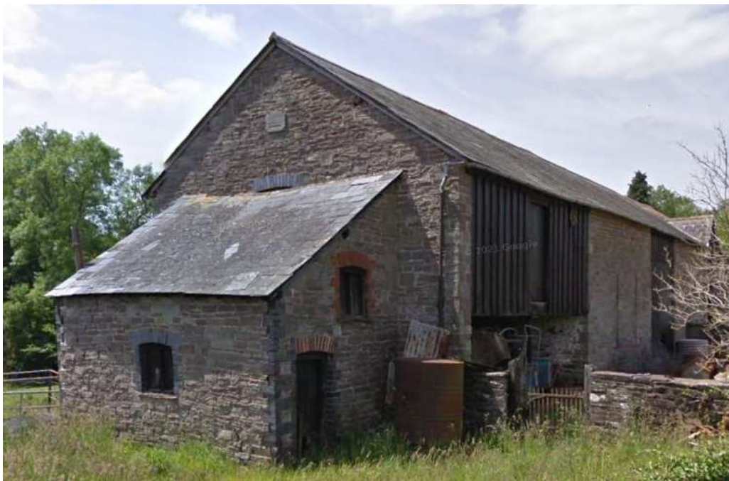
4. The east end with the fowl house and cart shed
