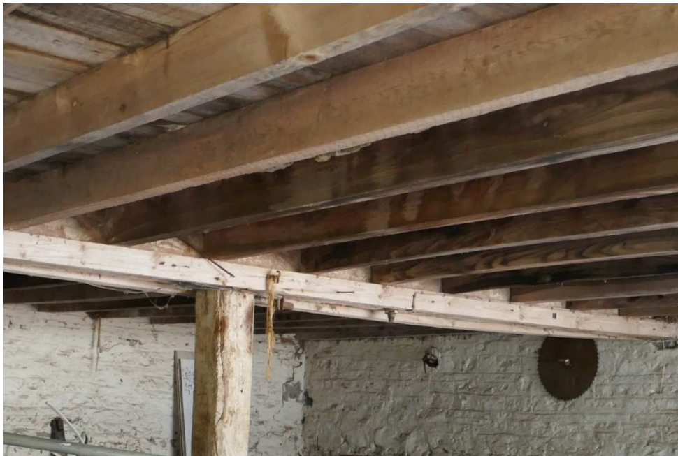
12. The patched structural timbers in the Cart Shed
