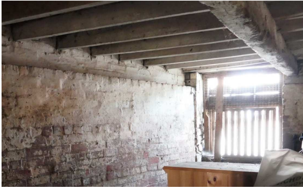
13. The beams and floor joists in the Cowhouse
