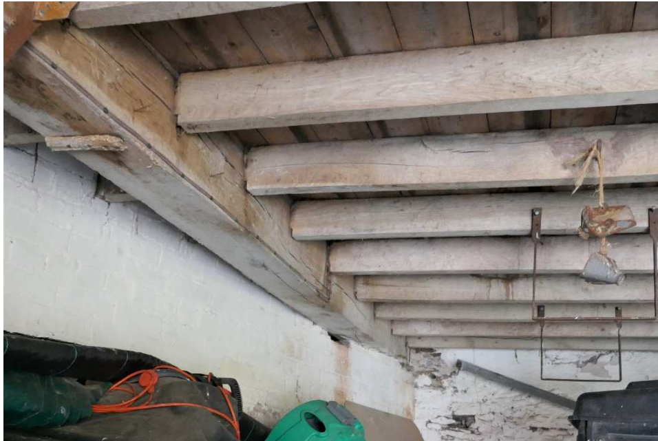
15. The floor joists and beams in the Cider House
