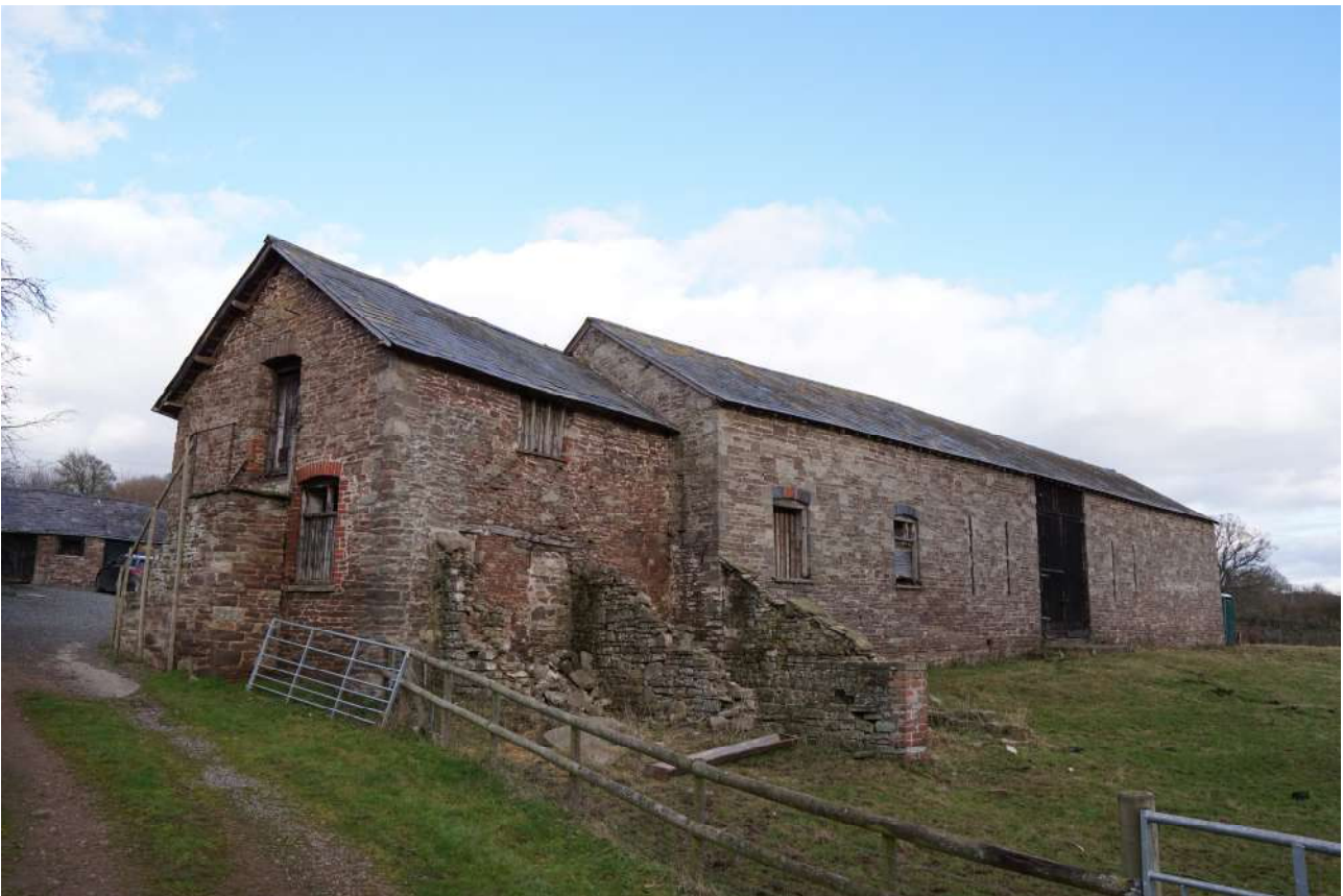
The view from the south-west. Cider House in foreground.
