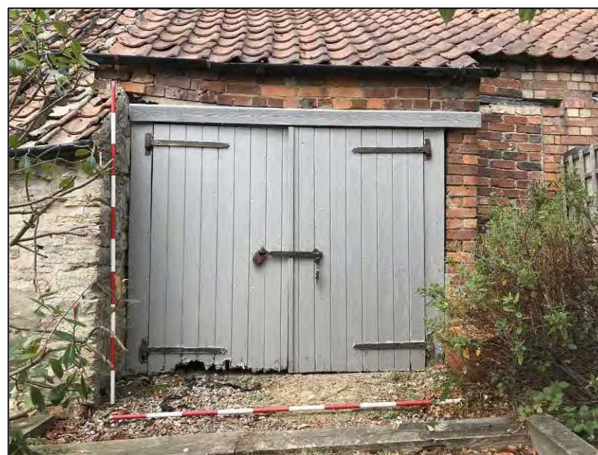
5. Cart entrance to outbuilding 2. Facing W
