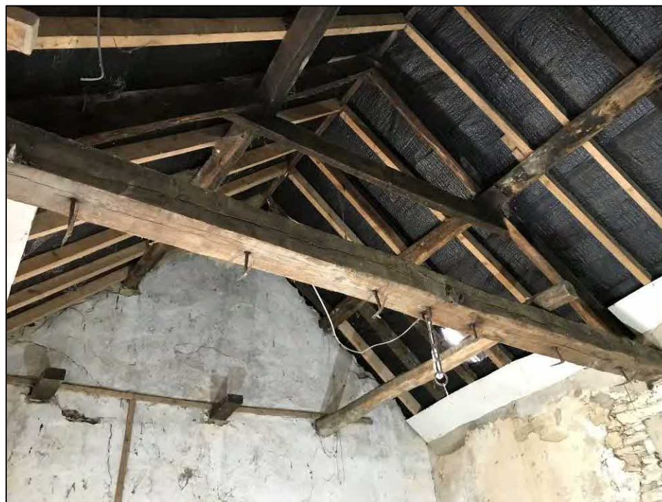
22. Outbuilding 1 interior: roof frame. Facing NE
