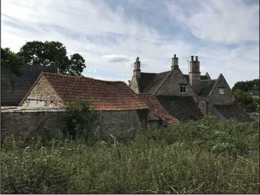
16. Overview of outbuildings. Facing SE
