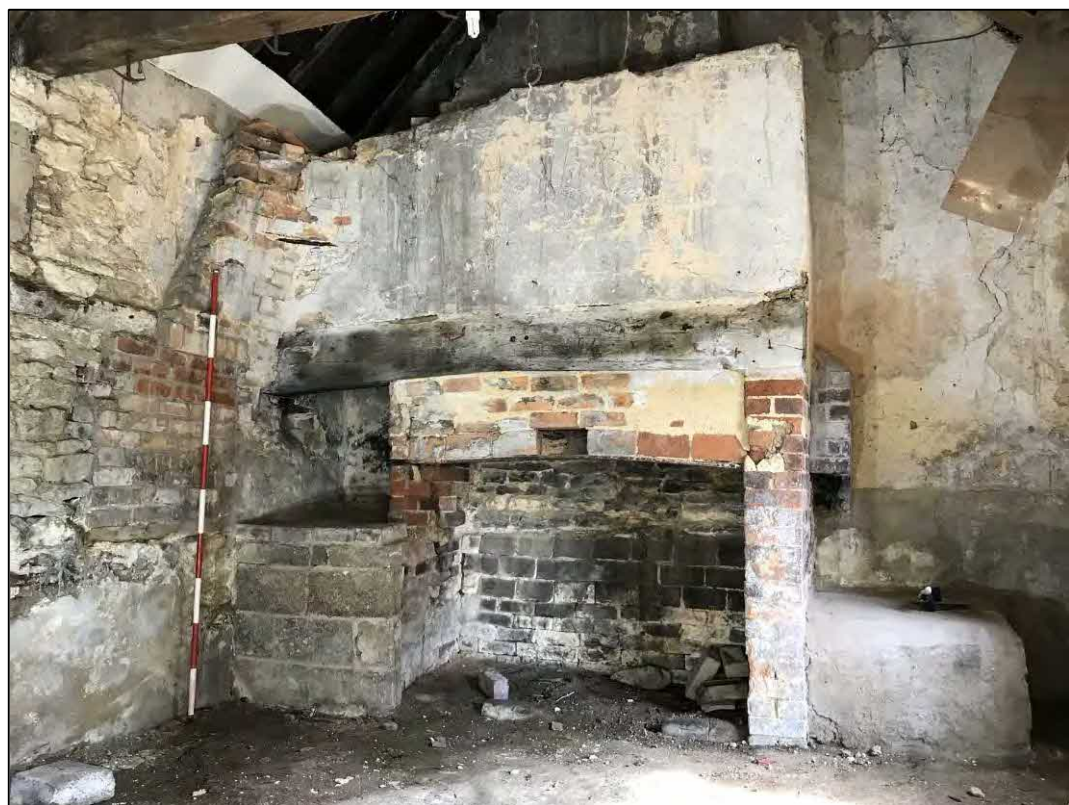
26. Outbuilding 1 interior: fireplace and chimney breast. Facing N
