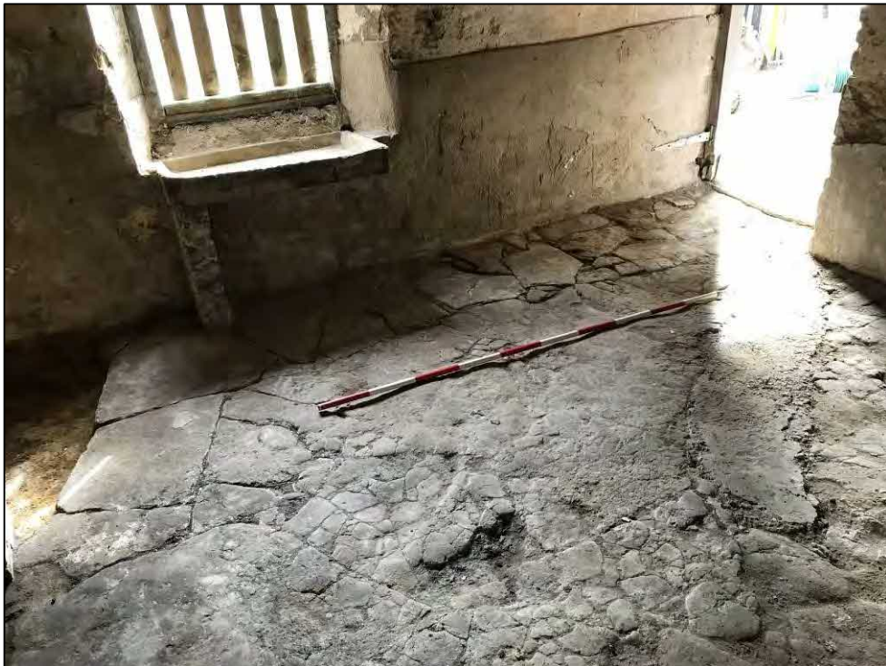
58. Outbuilding 1: limestone floor slabs after cleaning. Facing SW
