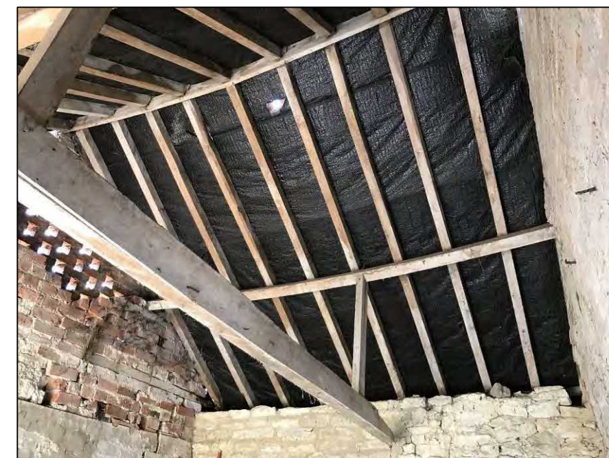
41. Outbuilding 2 interior: roof structure. Facing SW
