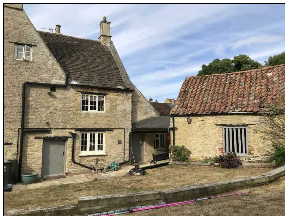
2. Outbuilding 1 and Home Farm House. Facing SW
