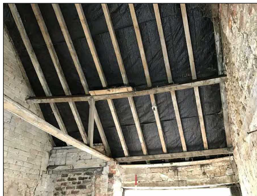
40. Outbuilding 2 interior: roof structure. Facing NE
