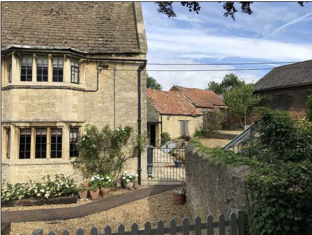
20. Southeast elevation of Home Farm House with outbuildings in the background. Facing NW
