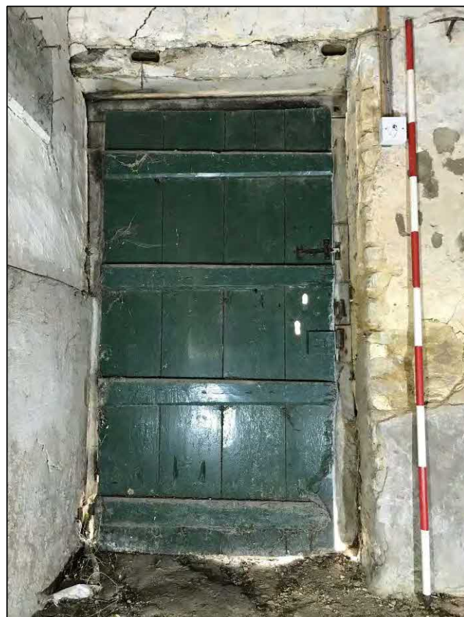
29. Outbuilding 1 interior: plank and batten door. Facing S
