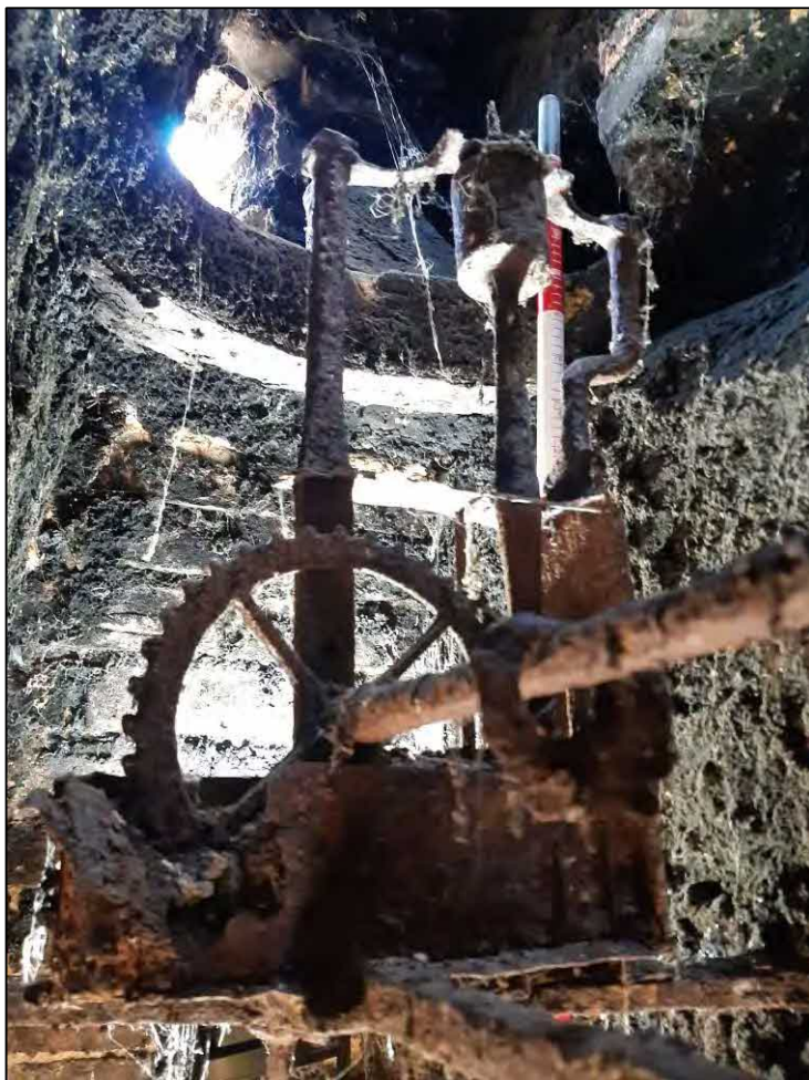
32. Outbuilding 1: chimney breast interior. Smoke jack mechanism (c. 18 th century)
