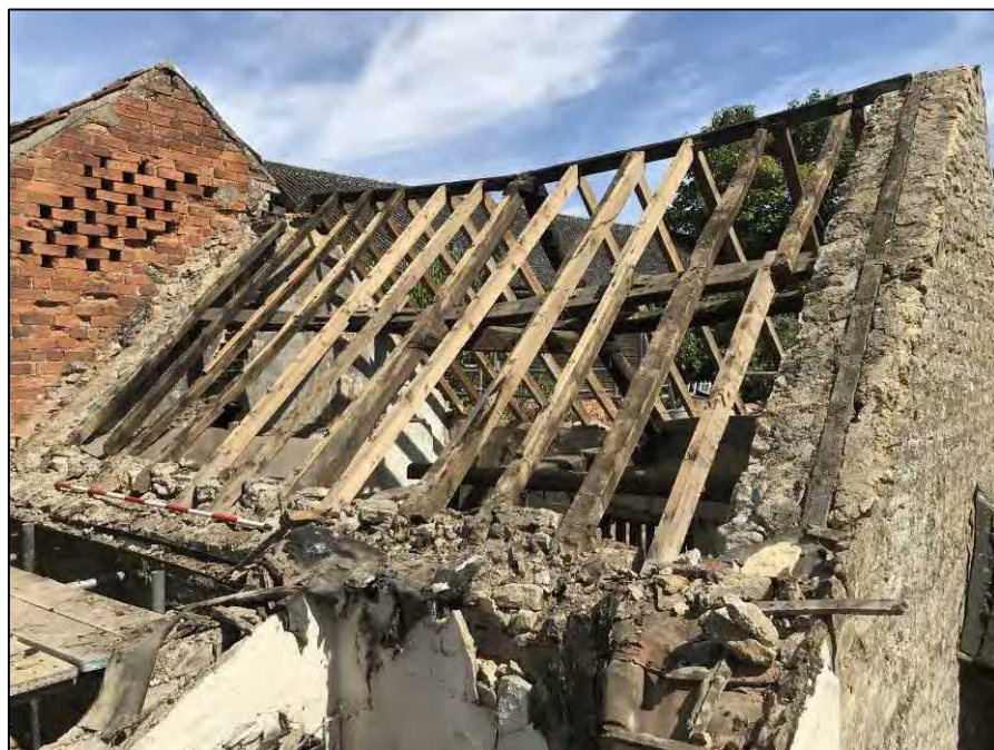
48. Outbuilding 1: roof structure. Facing NE
