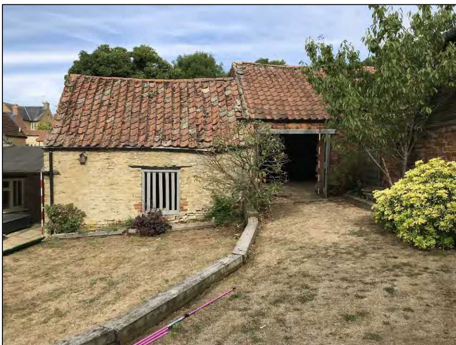
1. Overview of outbuildings. Facing W
