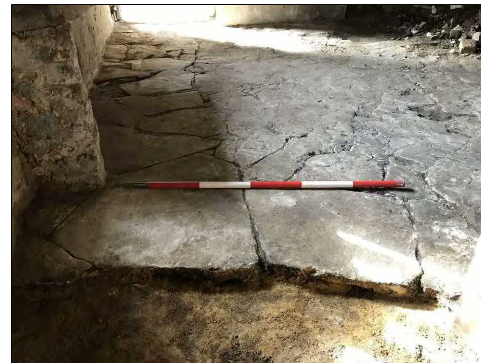
60. Outbuilding 1: limestone floor slabs after cleaning. Facing S
