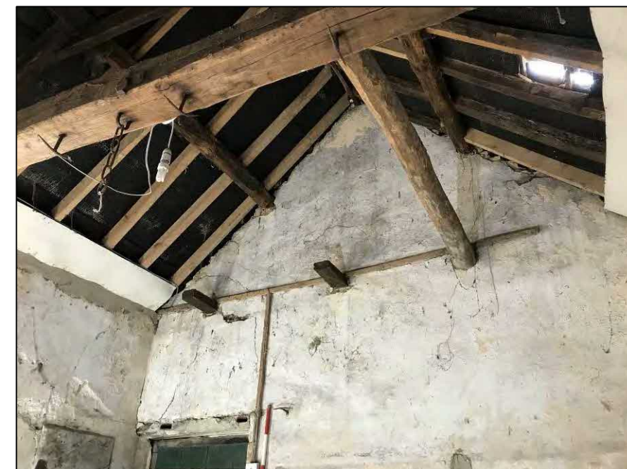
23. Outbuilding 1 interior: roof frame. Facing S
