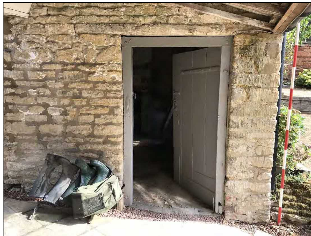
8. Doorway to outbuilding 1. Facing N
