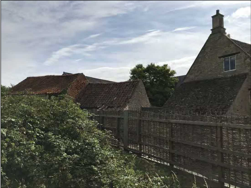
12. Overview of outbuildings. Facing NE
