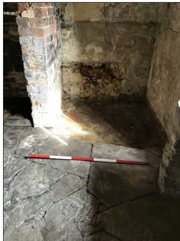
59. Outbuilding 1: limestone floor slabs above bedrock. Facing N
