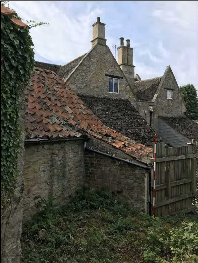
14. West elevation of outbuilding 1. Facing S
