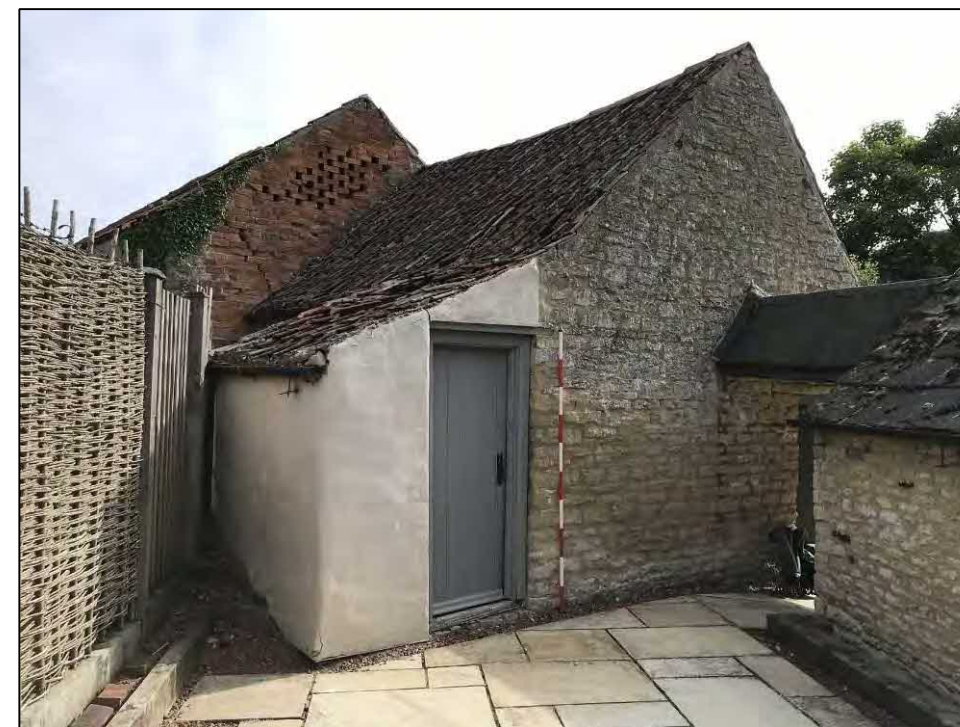
6. Doorway to WC. Facing NE
