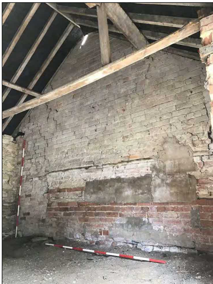
36. Outbuilding 2: internal north elevation. Facing N
