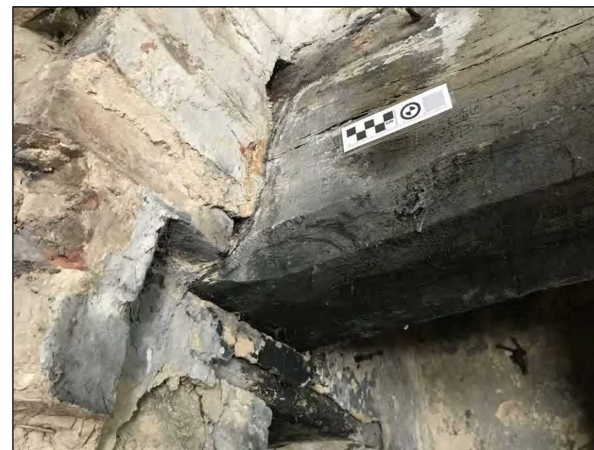
31. Outbuilding 1 interior: detail of chamfered lintel beam in fireplace. Facing NE
