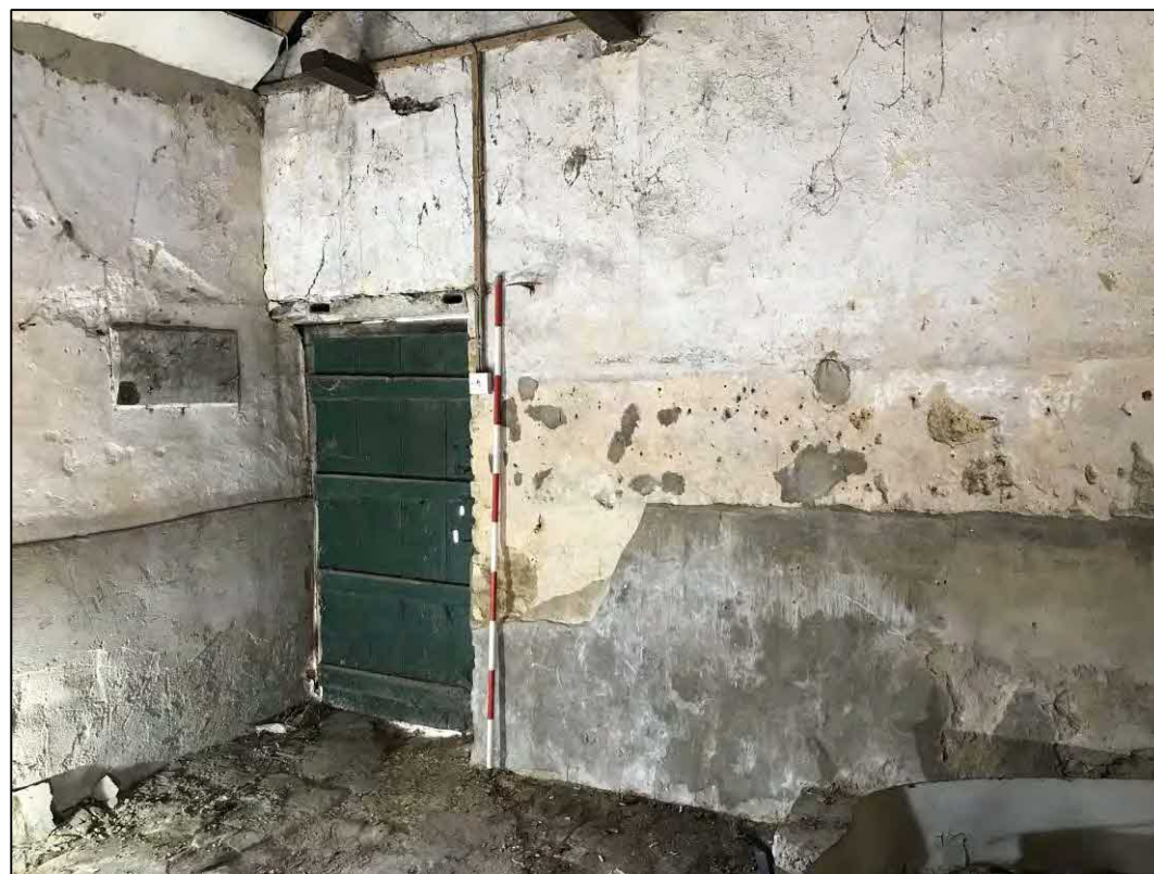
30. Outbuilding 1: internal south elevation. Facing SE
