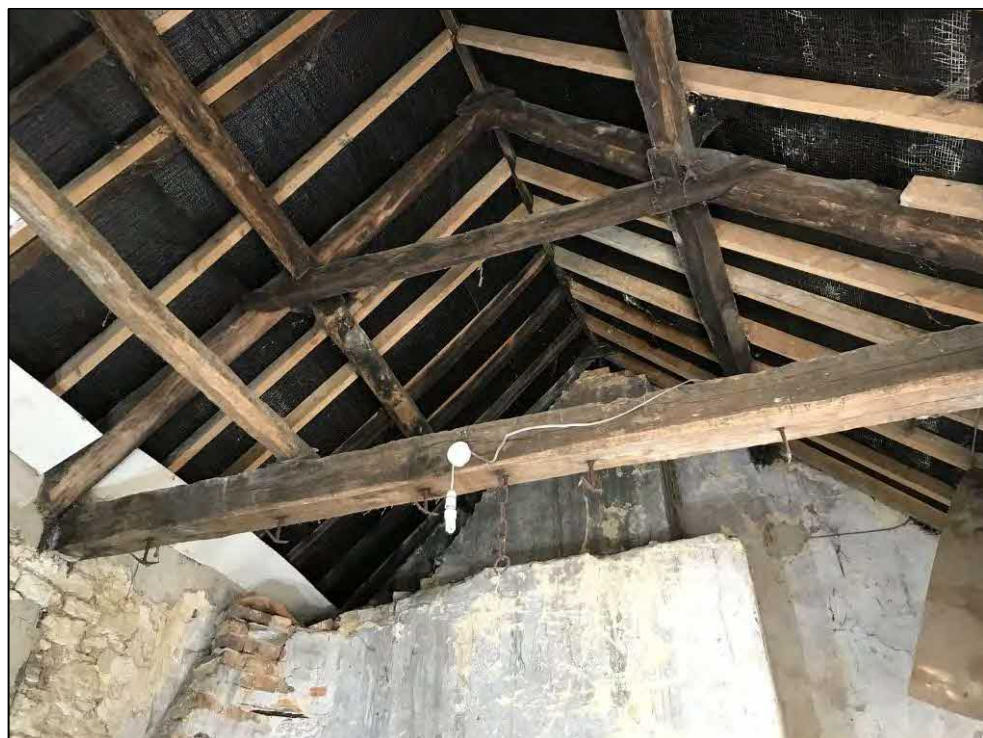
21. Outbuilding 1 interior: roof frame. Facing N
