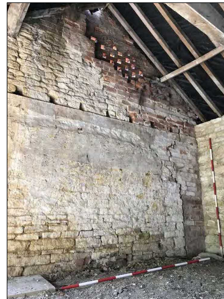
38. Outbuilding 2: internal south elevation. Facing SW
