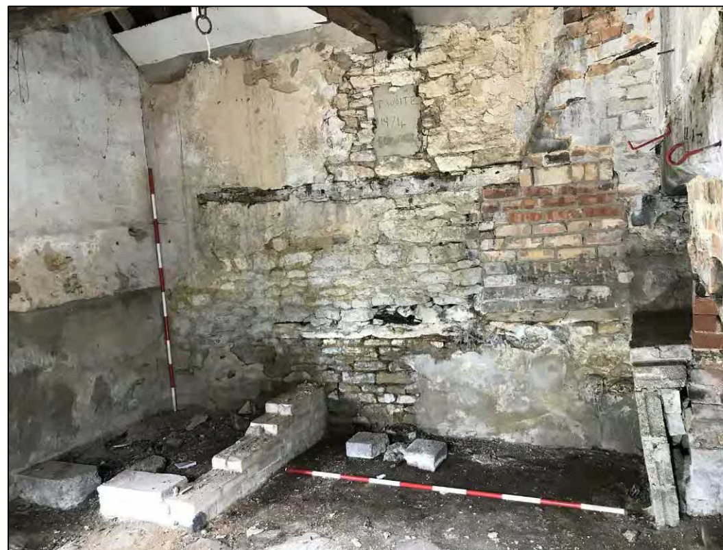
25. Outbuilding 1 interior. Facing W
