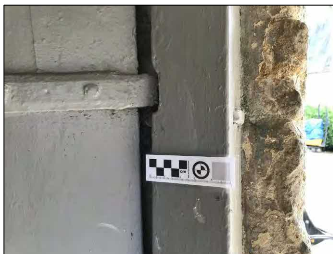
9. Detail of strap hinge/pintle fitting on doorway to outbuilding 1.
