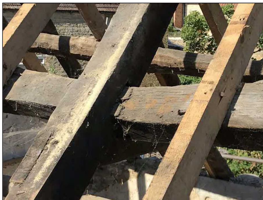
46. Outbuilding 1: principal rafter/ purlin joint
