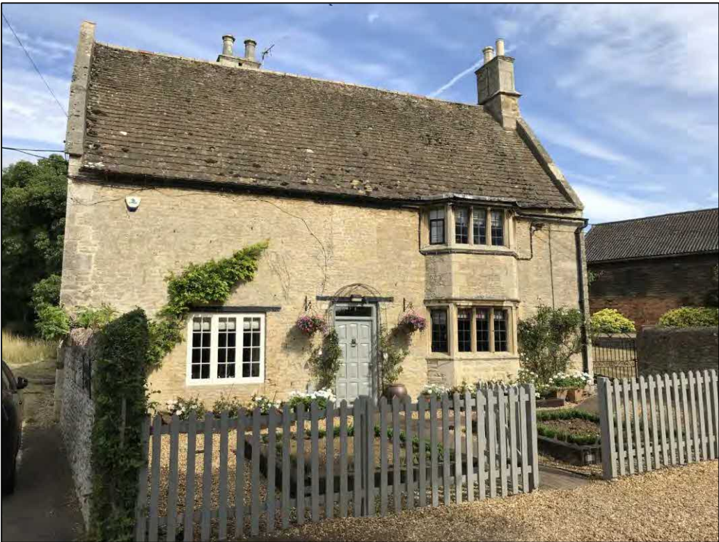
19. Southeast elevation of Home Farm House. Facing N
