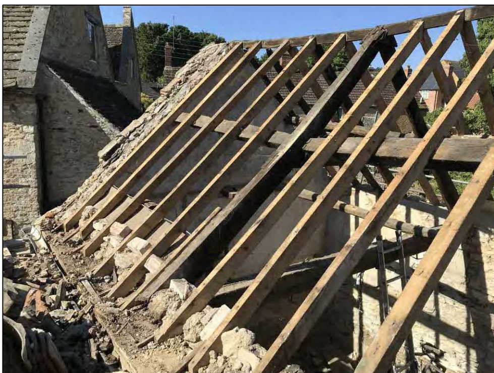
45. Outbuilding 1: roof structure. Facing SW
