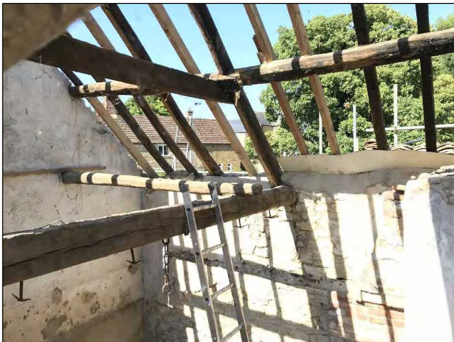
42. Outbuilding 1: roof structure. Facing W
