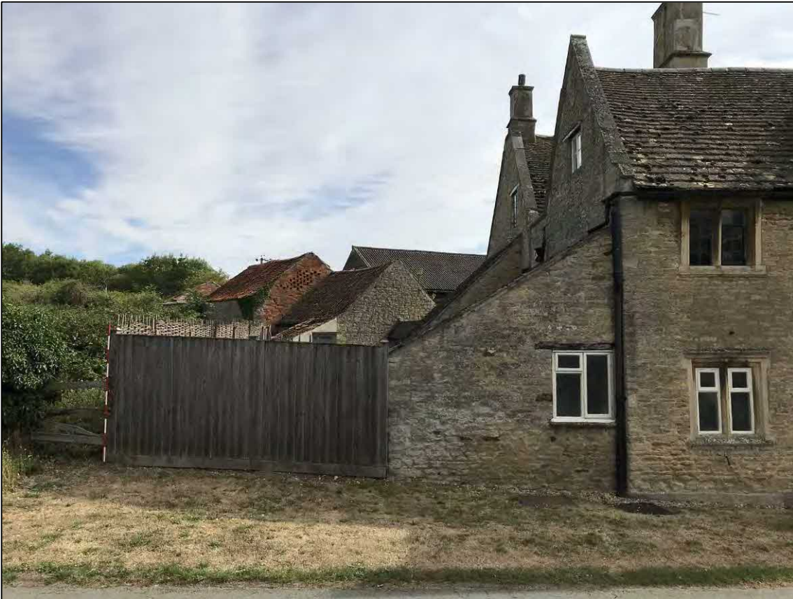
18. Southwest elevation of Home Farm House. Facing NE
