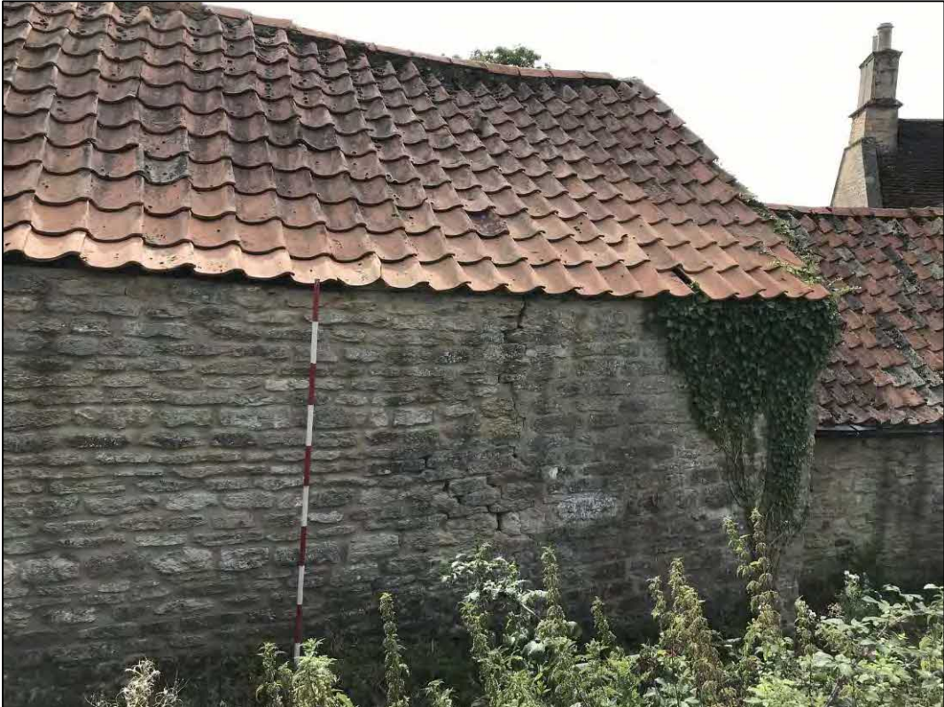
13. West elevation of outbuilding 2. Facing SE
