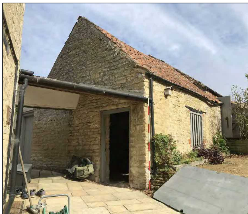
4. Doorway of outbuilding 1. Facing NW
