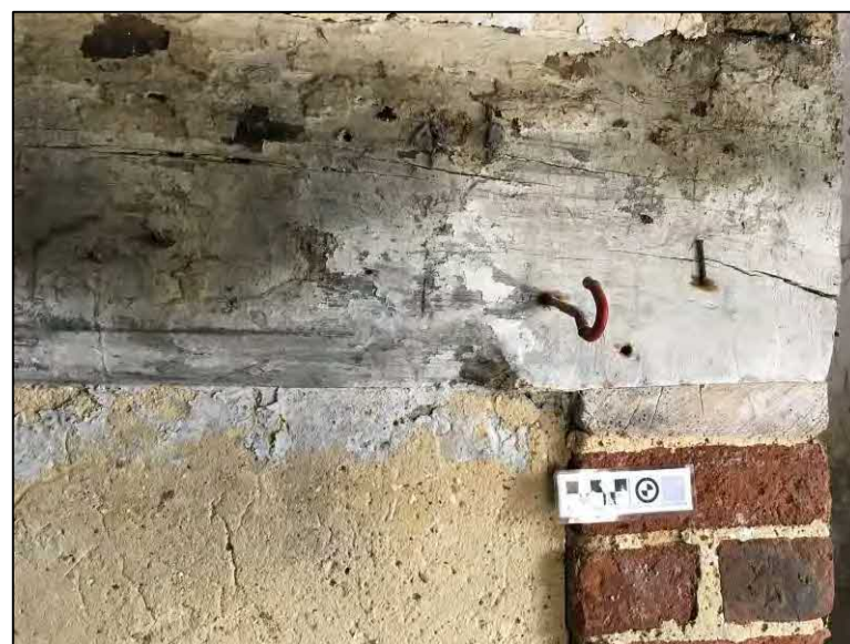
27. Outbuilding 1 interior: detail of chamfered lintel beam in fireplace. Facing N
