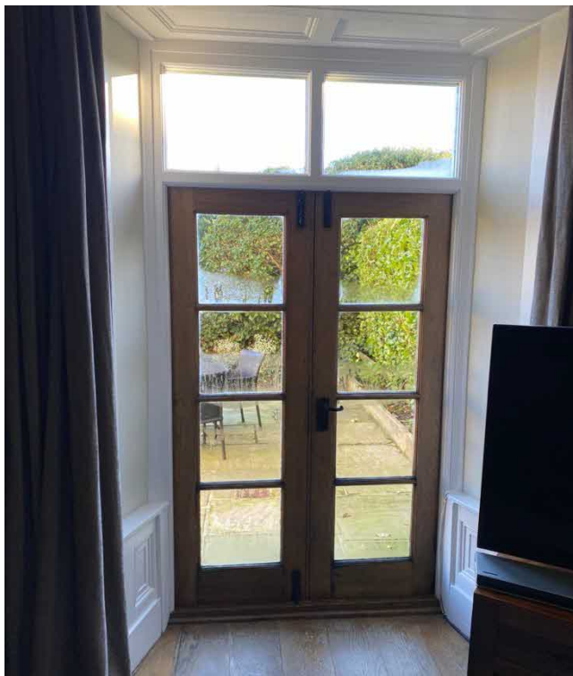
Inside view of patio door No 5 which include a window above. The window does not open, but both patio doors open on hinges.
