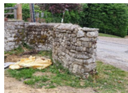
19 new stone wall replica to be built from existing reclaimed stones on site
