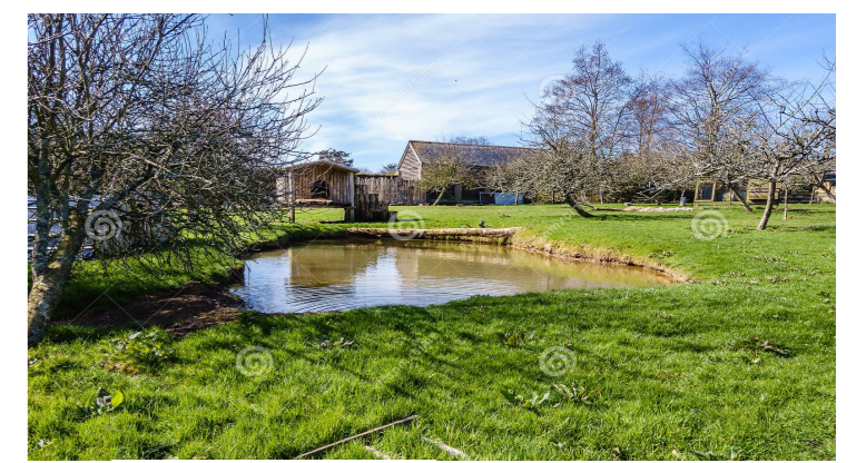
6 open rainwater pond
