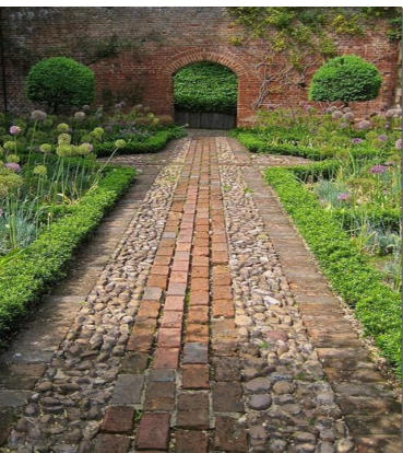
4 reclaimed brick and stone path
