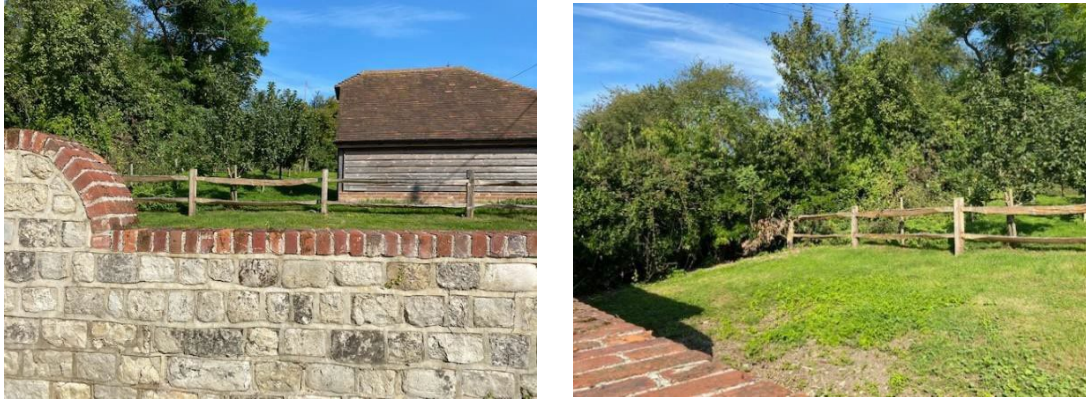
Existing boundary treatments to be replicated at the front and rear boundaries
