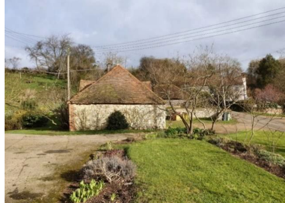
Barn South Elevation showing the change in level
