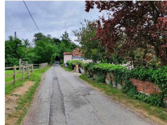
Court Lodge to the North and East of Vanity Lane
