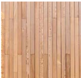
Timber Vertical Cladding
