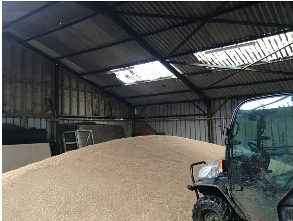
Plate 4: Building 1, interior (west section)
