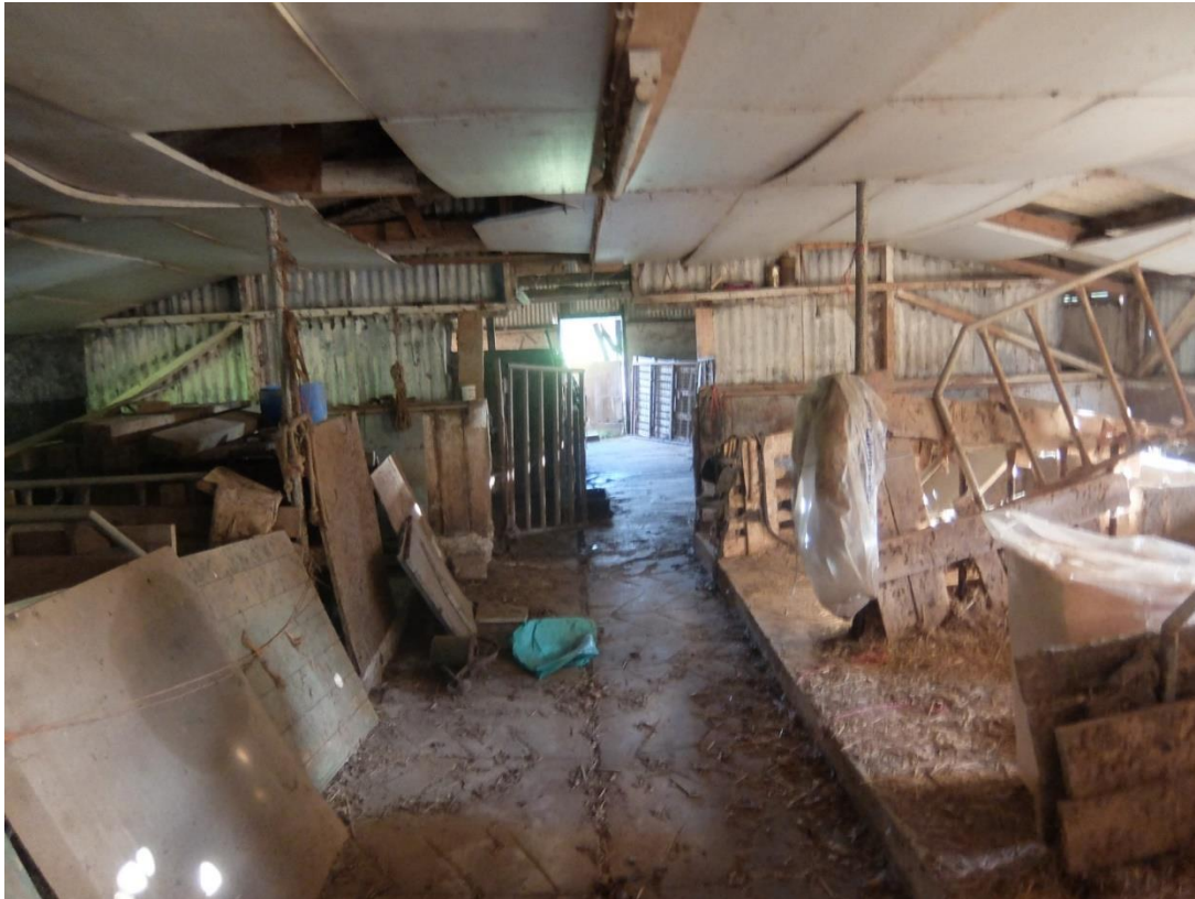
Internal view within second section from the right hand end
