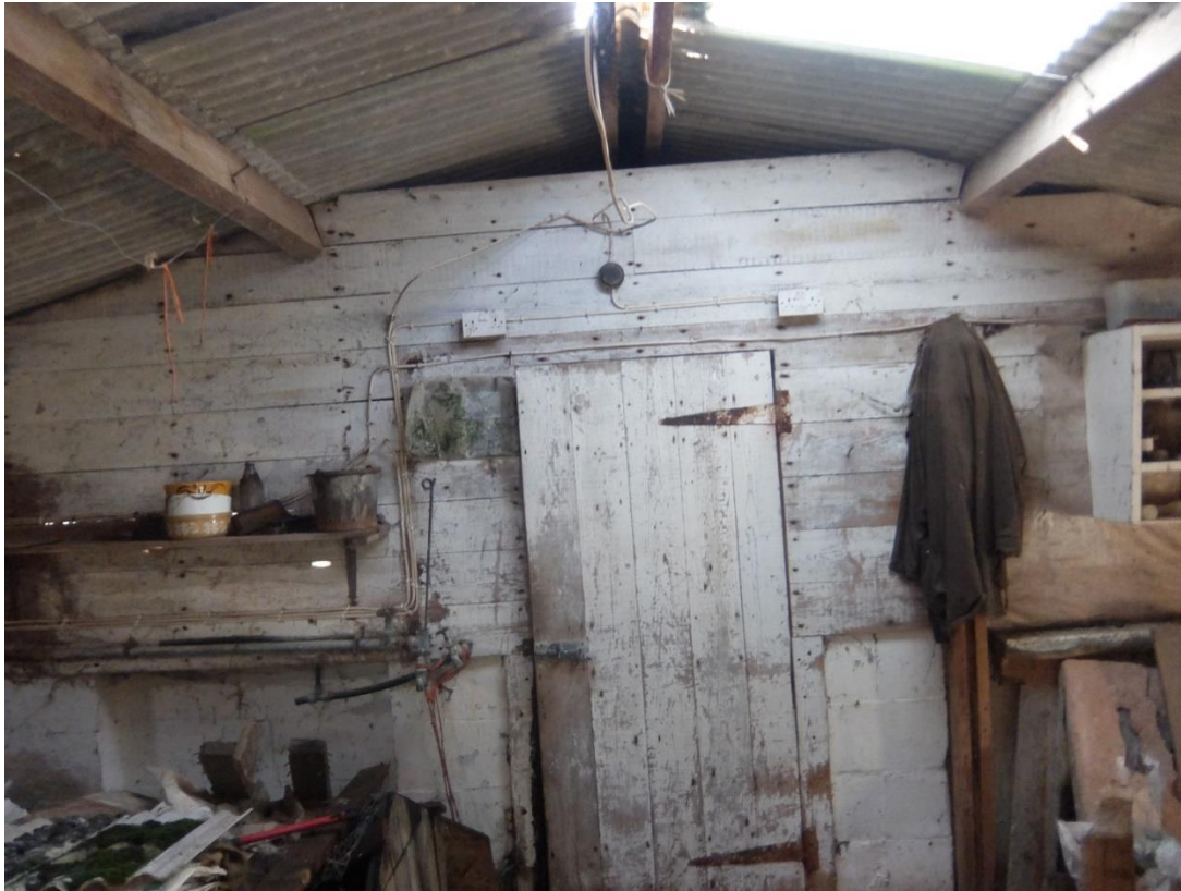
Internal view within fourth section from the right hand end
