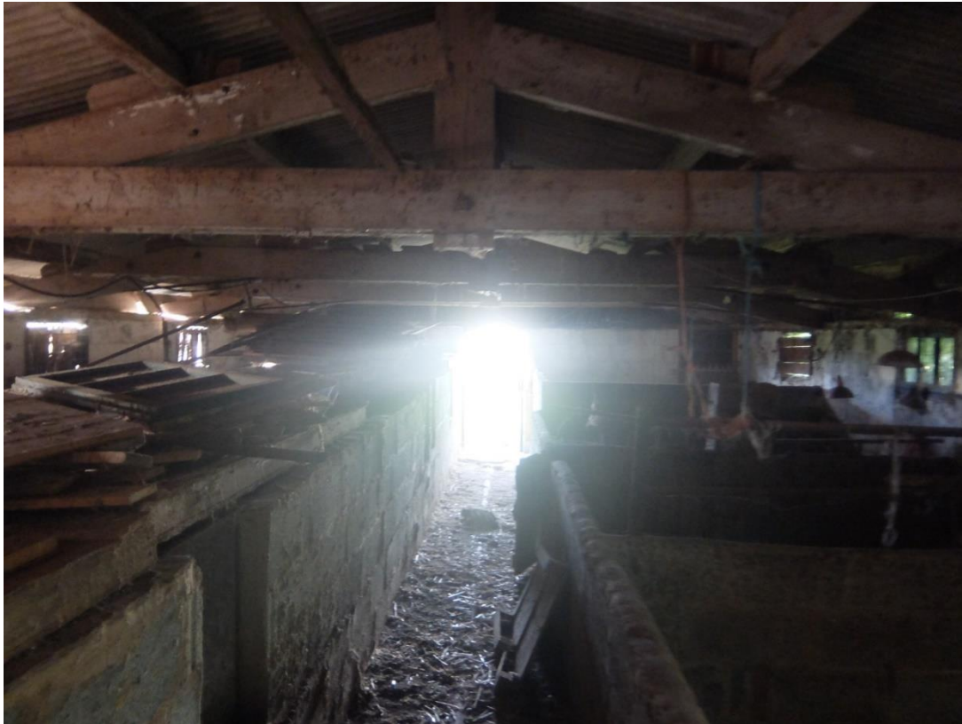
Internal view within left hand end section
