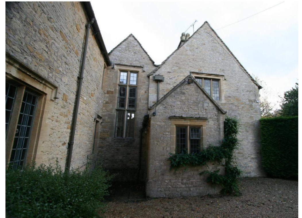
Internal (North West) elevation
