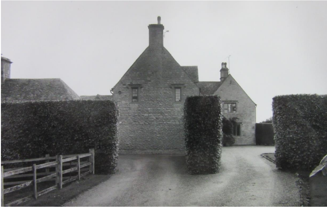
Figure 13: Rear north-west elevation of the farmhouse, 1991 (Historic England), illustrating the 1950s 2-storey extension to the north end of the service range.
