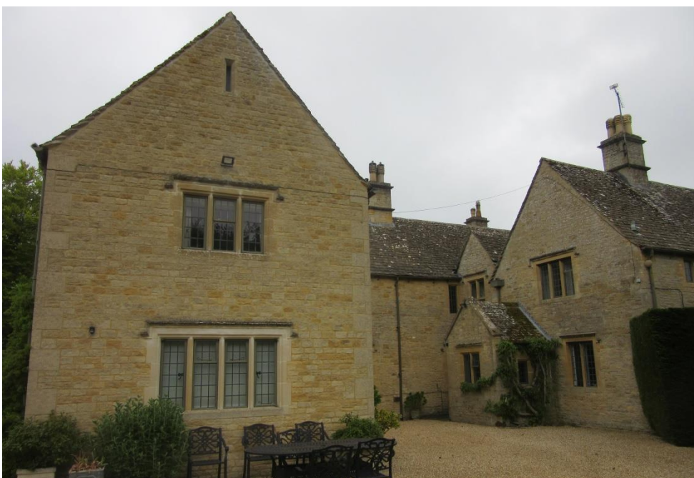
Figure 18: The "courtyard" created by the 1997 extension (left) with the 1958 porch and 1961 stair infill (centre).
