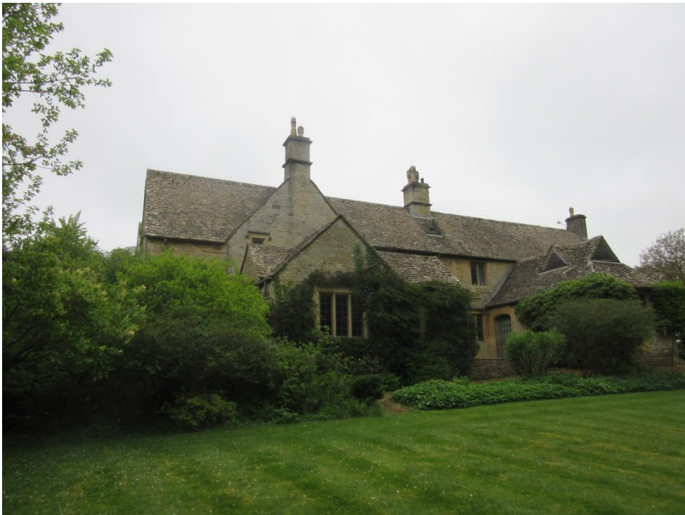
Figure 20: The side (north-east) elevation with the extended gables to the front elevation (left), 1970s single-storey extension (centre left) and original dairy (right).
