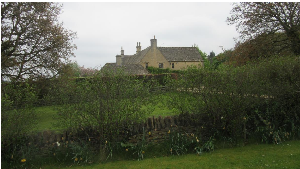
Figure 3: The farmhouse looks away from the farmstead, with the primary setting to the south-east.
