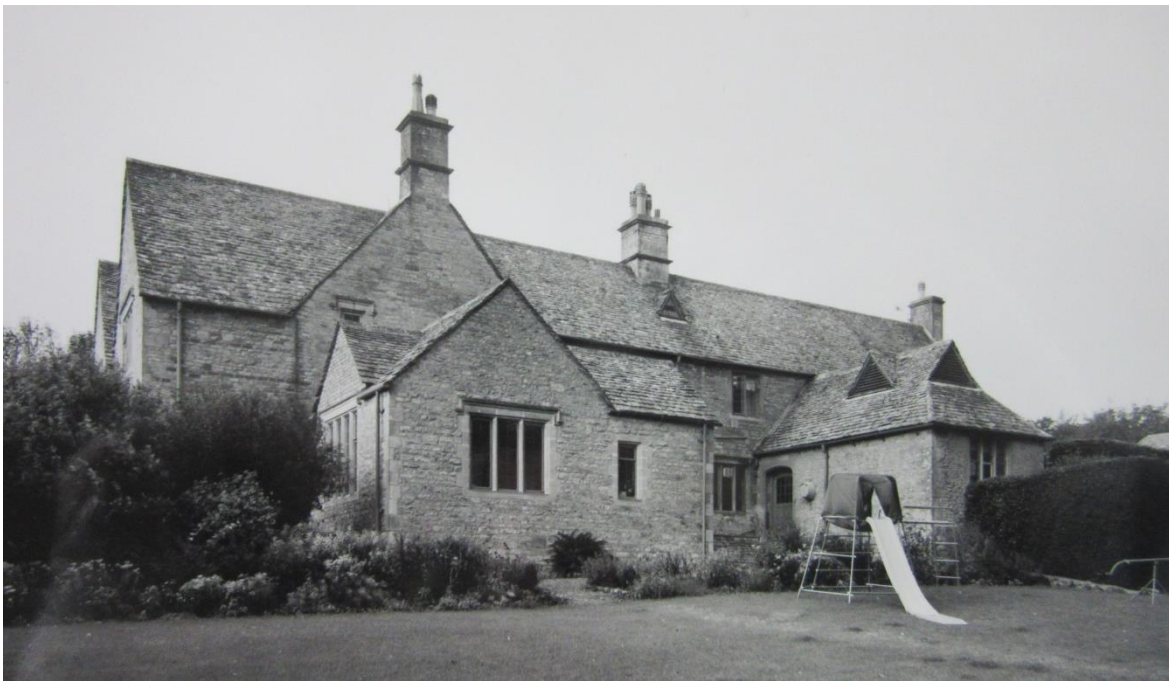
Figure 14: Side north-east elevation of the farmhouse, 1991 (Historic England), illustrating the late 1950s south-east extension and 1970s north-west side extension.
