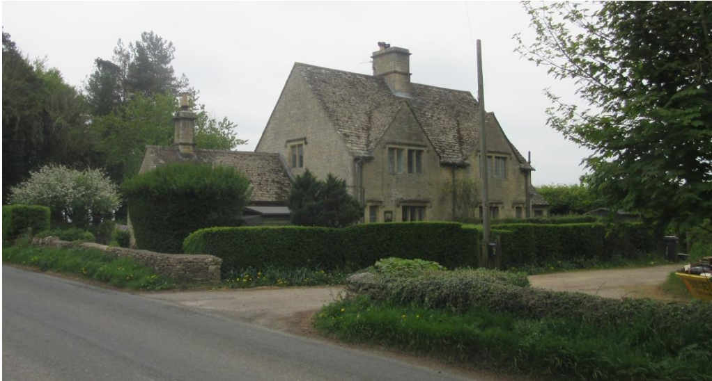
Figure 4a: Nos. 1 and 2 Manor Farm Cottages on the west side of Buckle Street.
