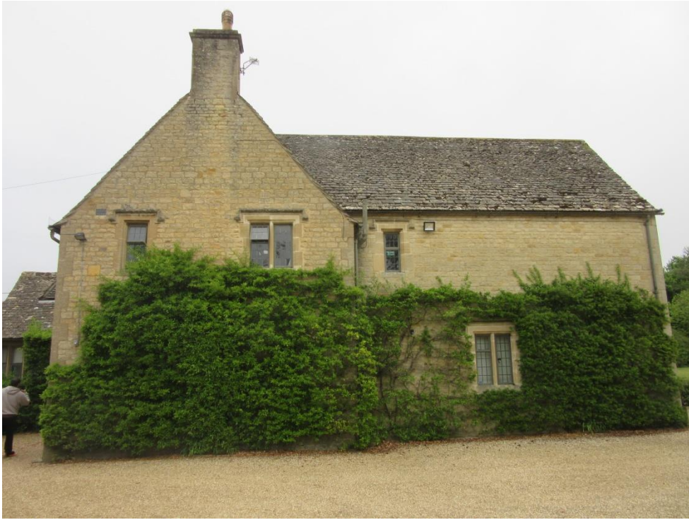
Figure 19: The rear north-west elevation showing the 1950s extension (left) and 1997 playroom extension (right).
