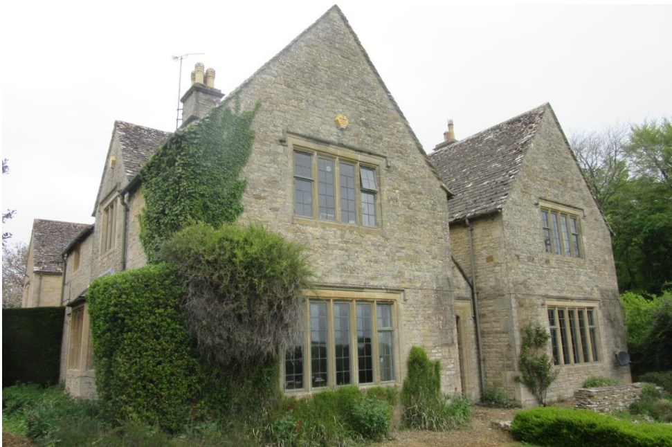
Figure 17: The front south-east elevation showing the extended gables.
