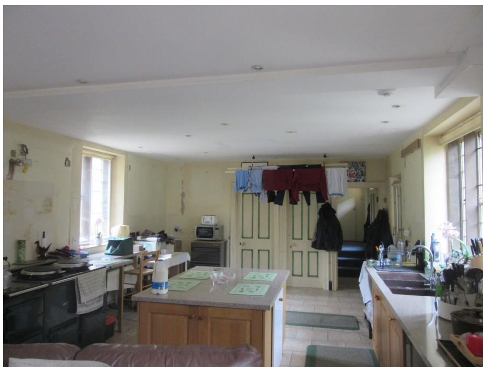
Figure 24: The kitchen occupies the original kitchen and scullery spaces with the insertion of a large steel joist to allow for the removal of the original central chimneybreast at an underdetermined date between 1961 and 1986.
