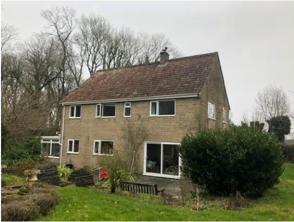
View of rear elevation
