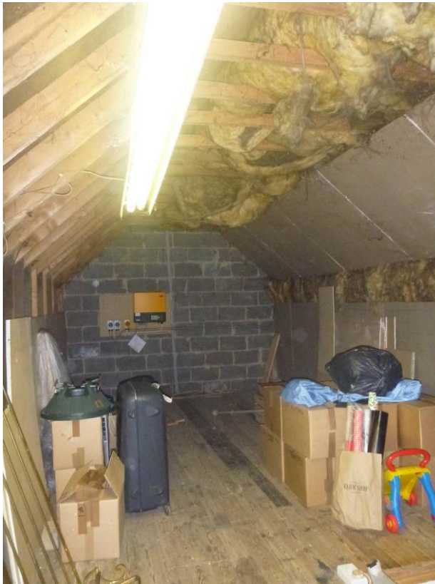
Fig 4: The loft space at Old Mill.
