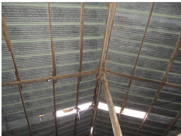
Photo 15: The roof had no features that might be occupied by bats
