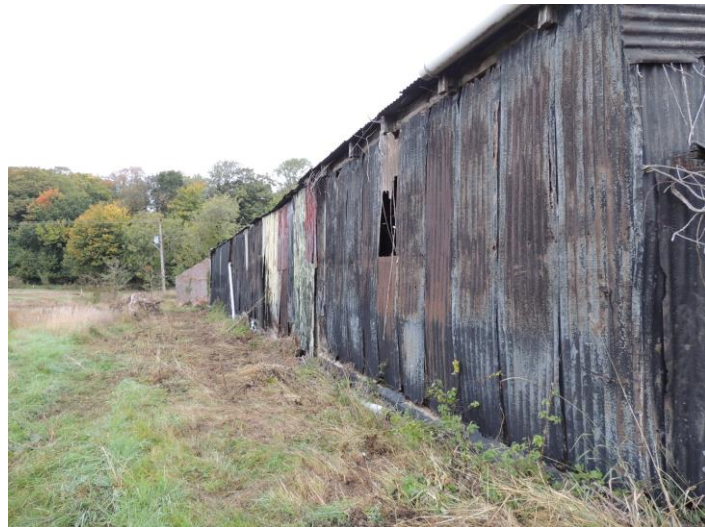
Photo 6: Looking northwards along western elevation
