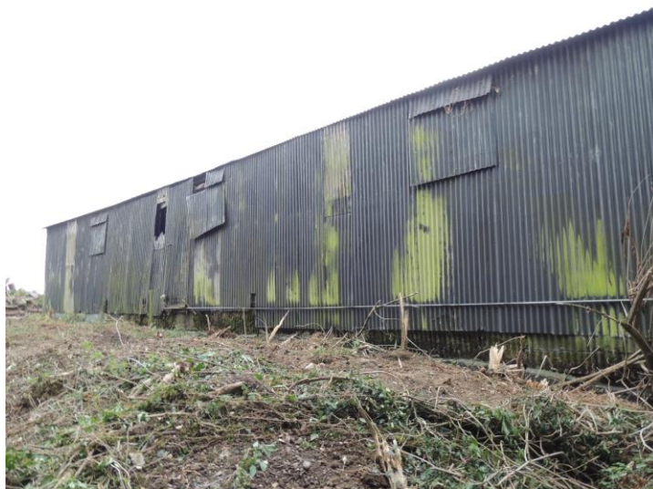
Photo 3: Part of eastern elevation
