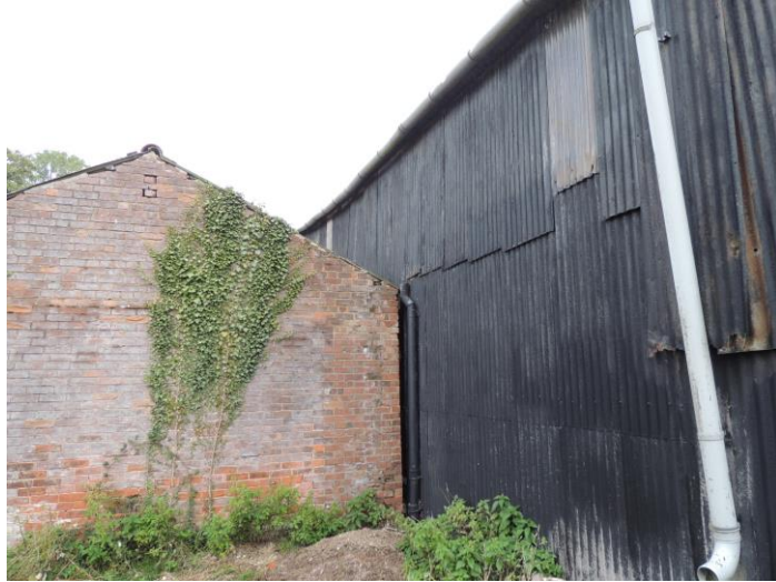
Photo 8: NW corner. The brick building is to be retained
