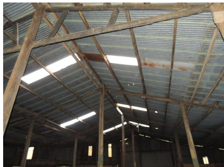
Photo 16: The roof had no features that might be occupied by bats
