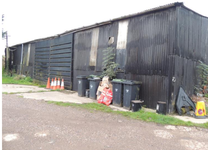
Photo 2: Part of eastern elevation
