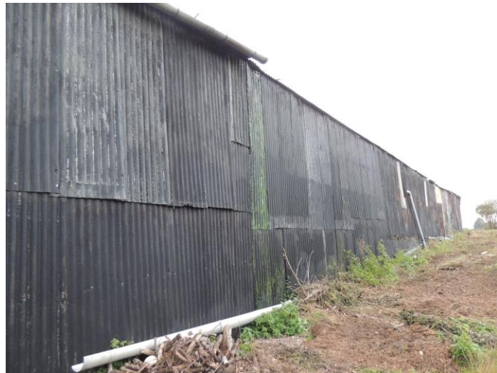
Photo 7: Looking southwards along western elevation
