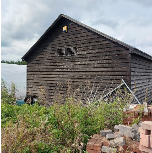
The timber clad existing agricultural barn.
