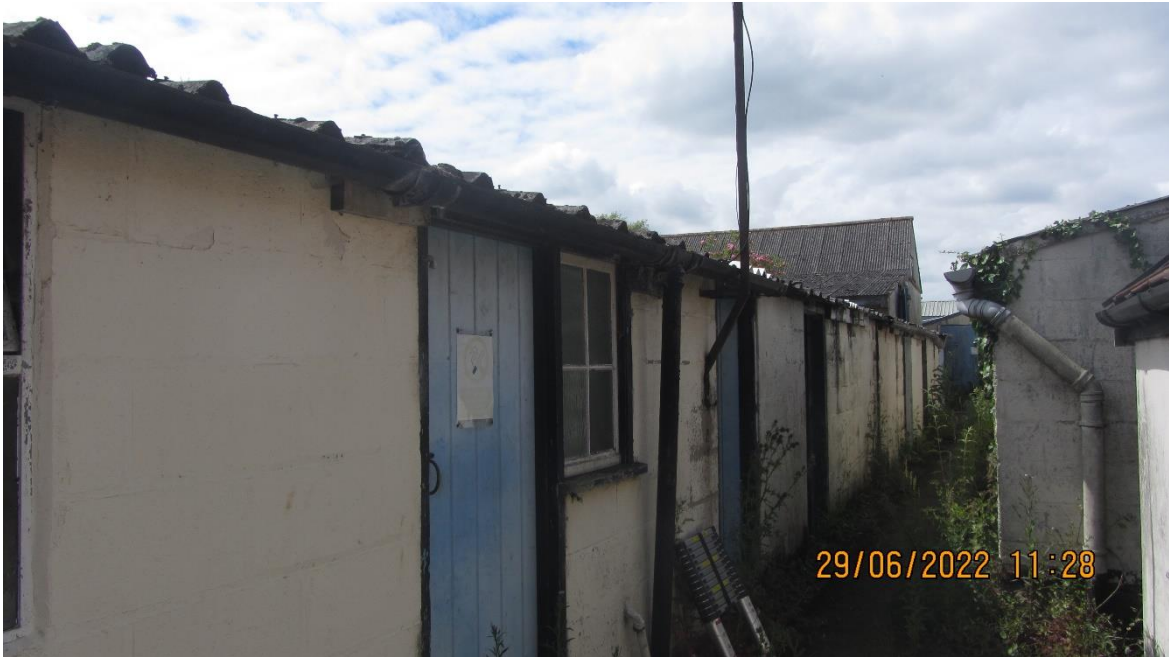
Photo 5: View west of exterior of Building 3
