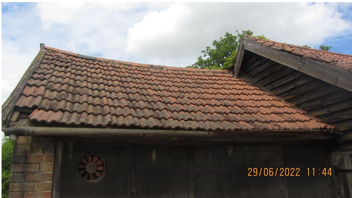
Photo 11: View north of exterior of Building 5
