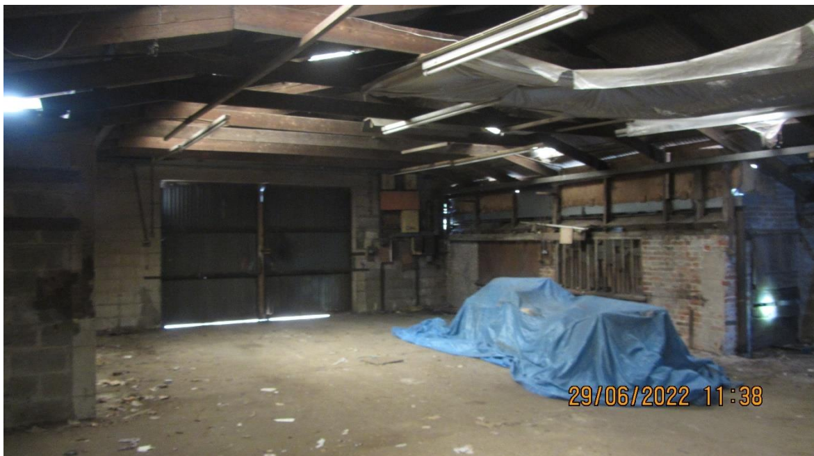
Photo 8: View of interior of Building 4
