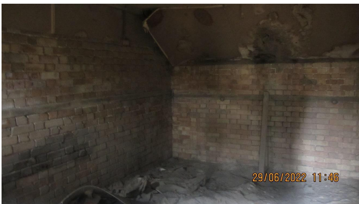
Photo 12: View of Building 5 interior
