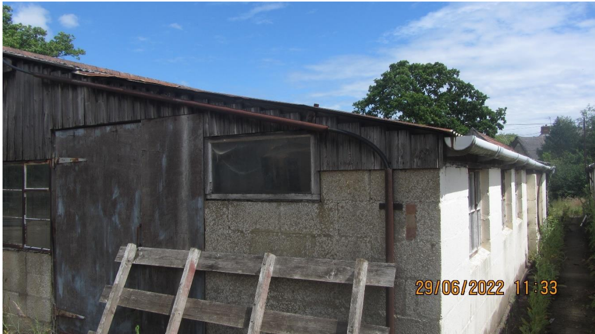
Photo 7: View east of exterior of Building 4
