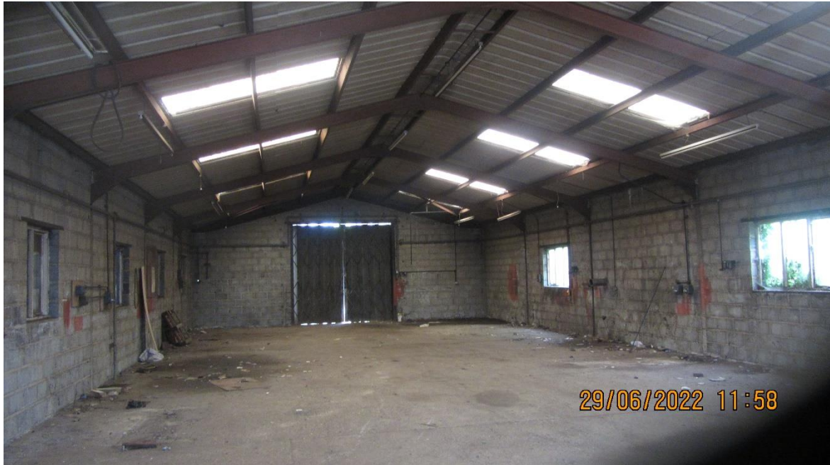
Photo 15: View of Building 6 interior
