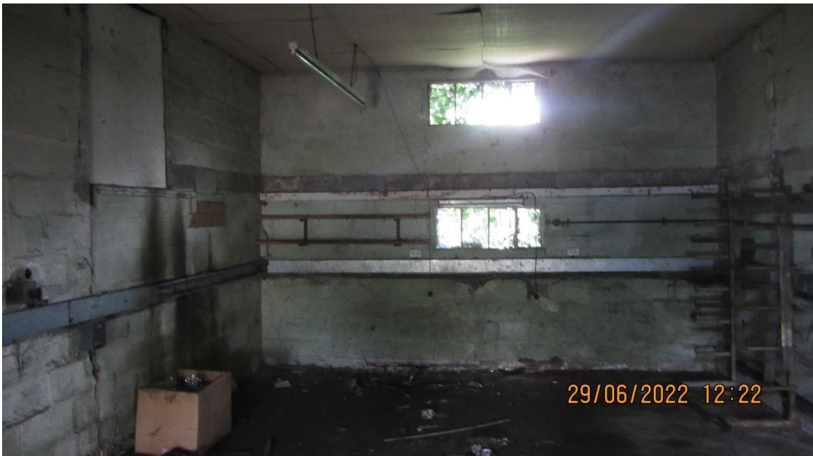
Photo 20: View of interior of Building 9
