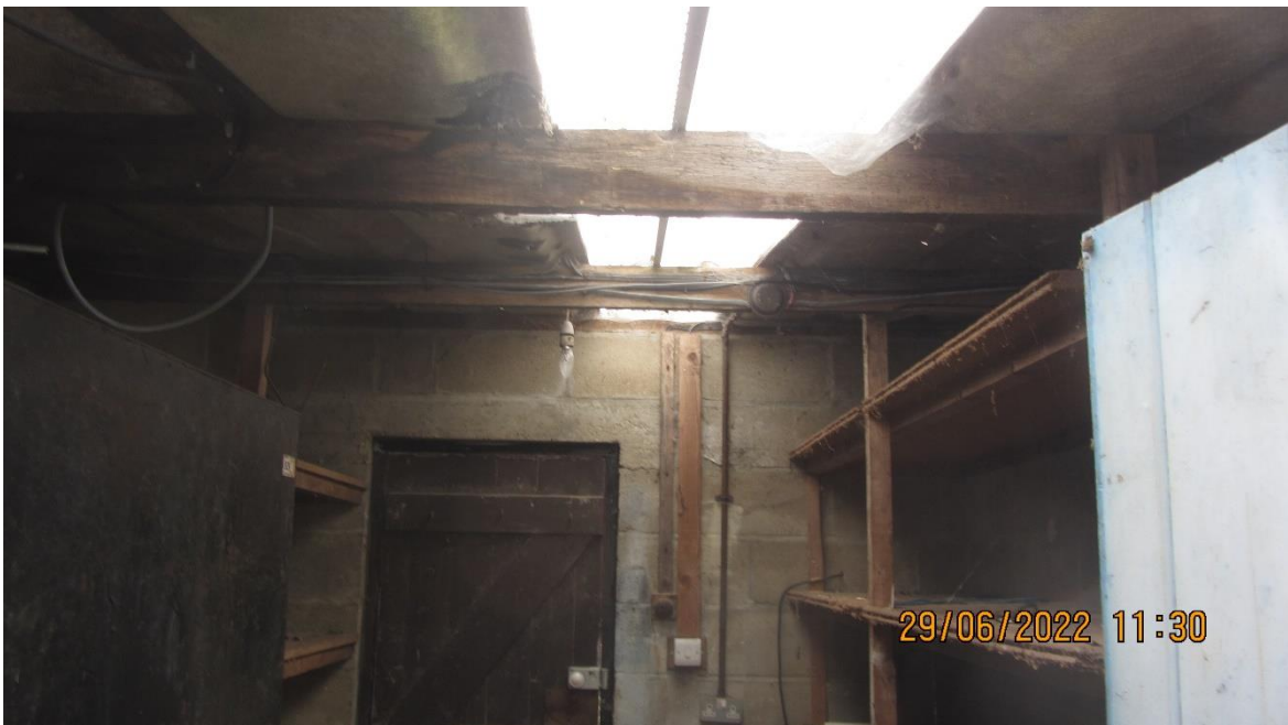
Photo 6: View of interior of Building 3
