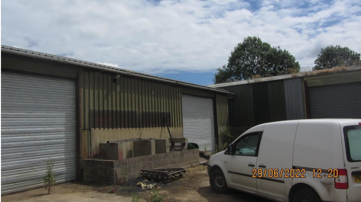
Photo 17: View east of Building 8 exterior
