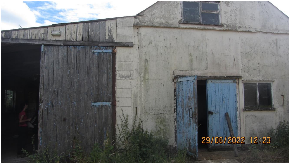
Photo 19: View south of Building 9 exterior
