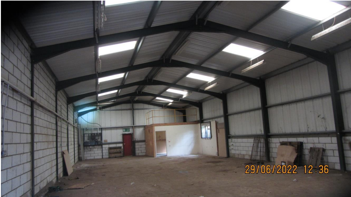
Photo 23: View of Building 11 interior
