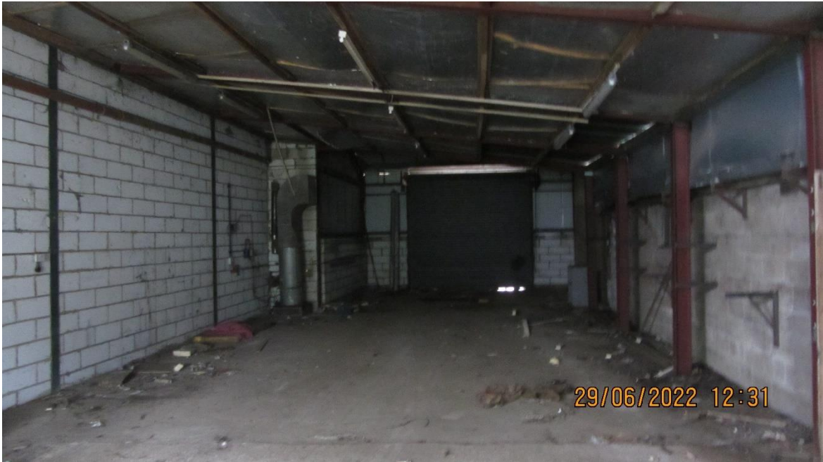
Photo 21: View of interior of Building 10
