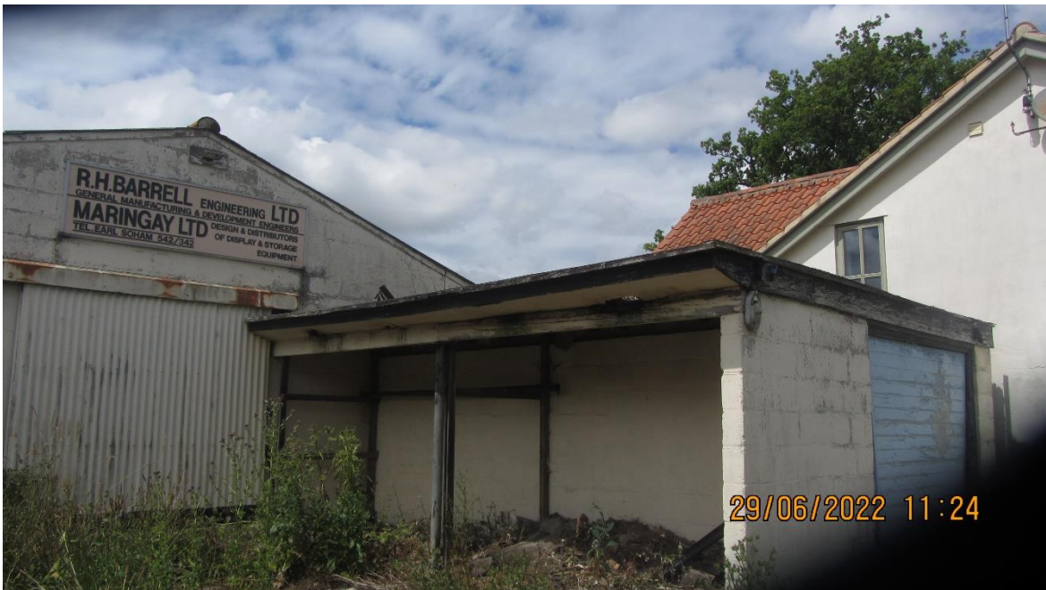
Photo 4: View north of exterior of Building 2
