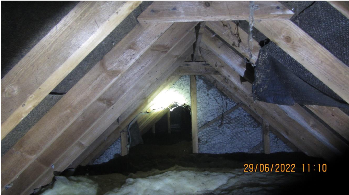
Photo 3: View of shallow loft void within Building 1
