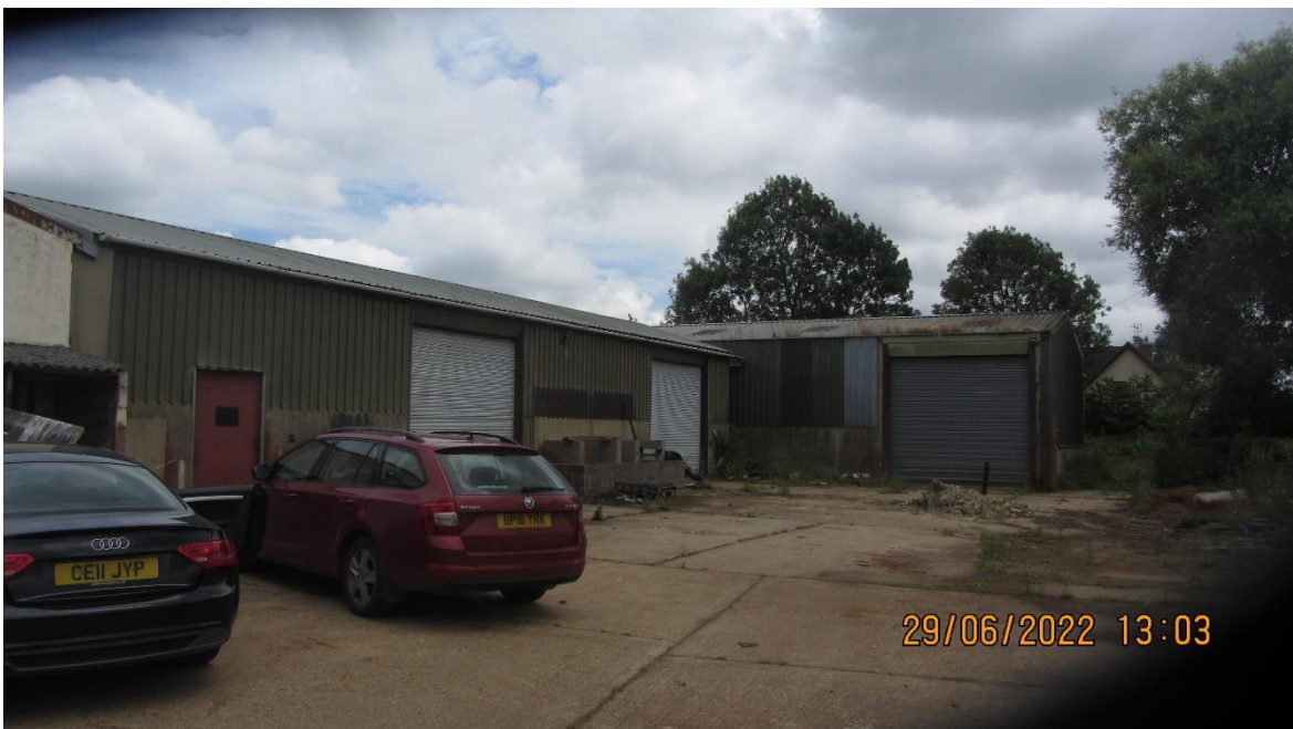
Photo 22: View south of exterior of Building 11 (on the right)
