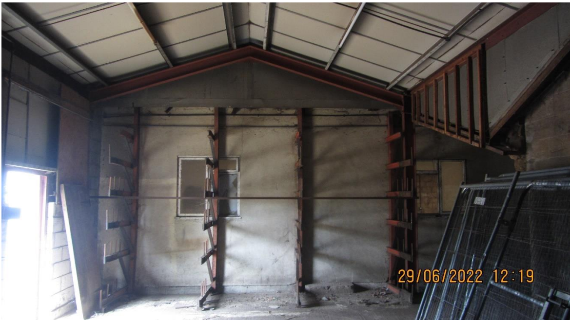
Photo 18: View of Building 8 interior
