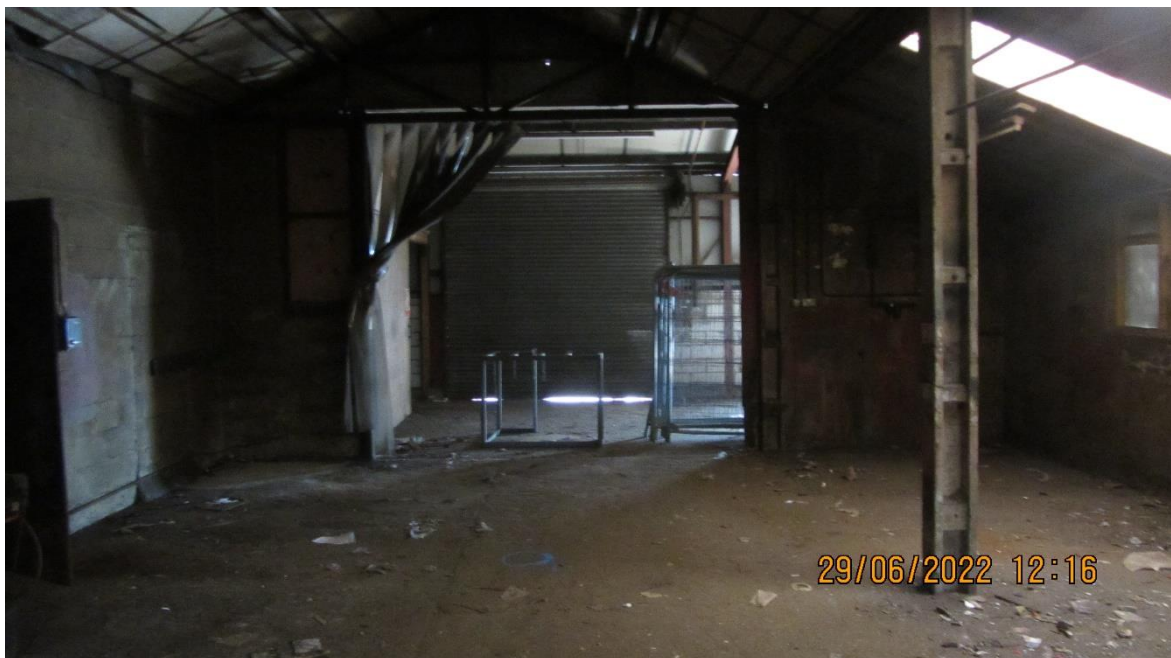
Photo 16: View of Building 7 interior
