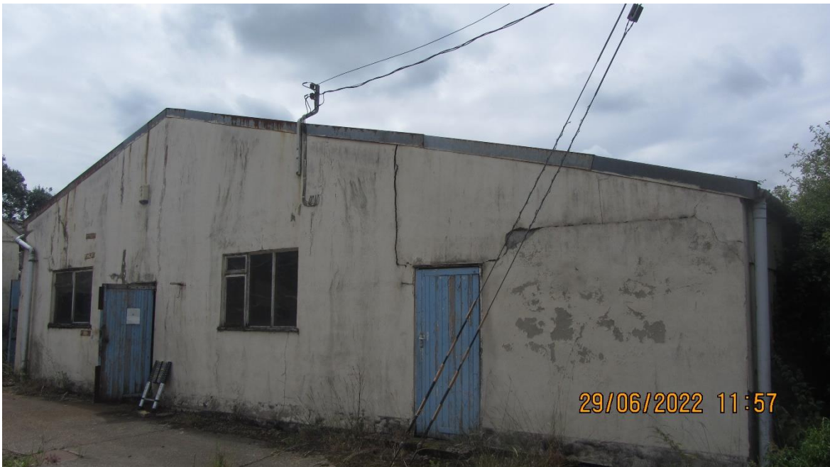
Photo 14: View west of Building 6 exterior
