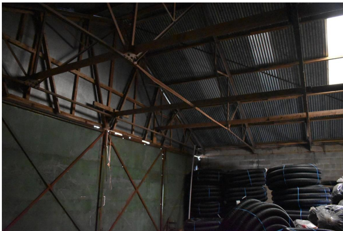
Photo 6 – Interior of Building 2
