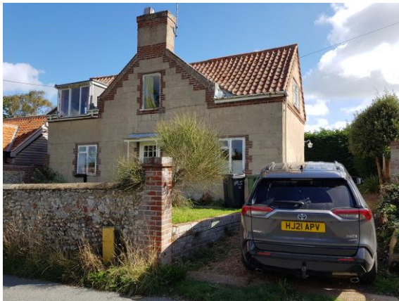
Fig 1: View of Victoria Cottage from Gong Lane
