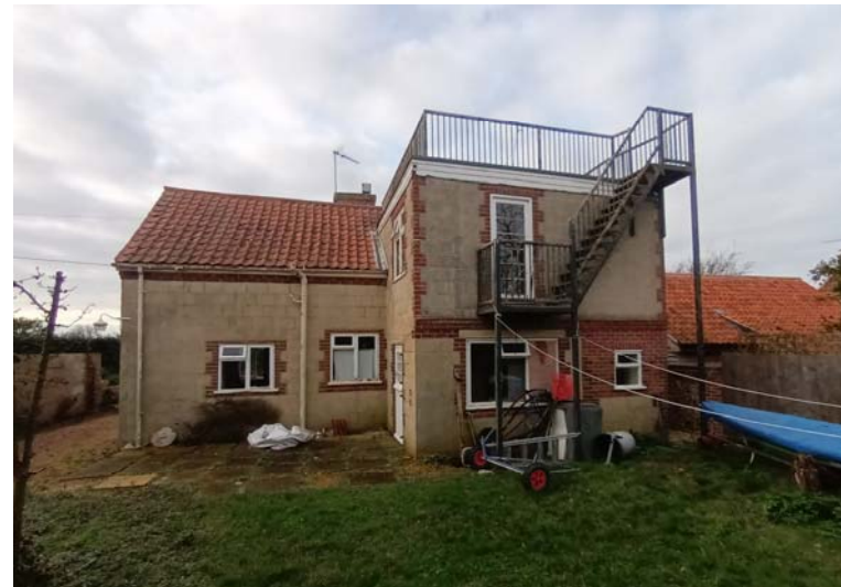
Photograph – existing east elevation
