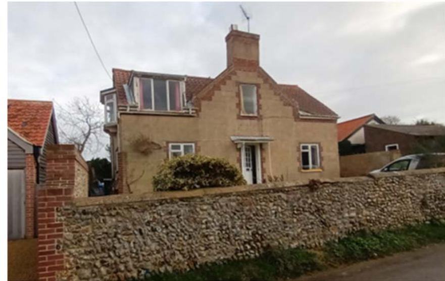
Photograph – Existing Property, Victoria Cottage (west elevation)
