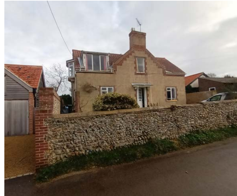
Photograph – Existing Property, Victoria Cottage (west elevation)
