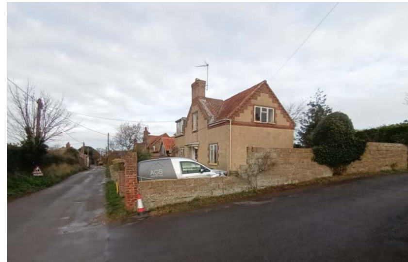
Photograph – Existing Property, Victoria Cottage (west elevation)
