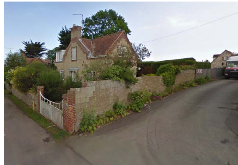
Google maps photograph 2011 (west elevation)
